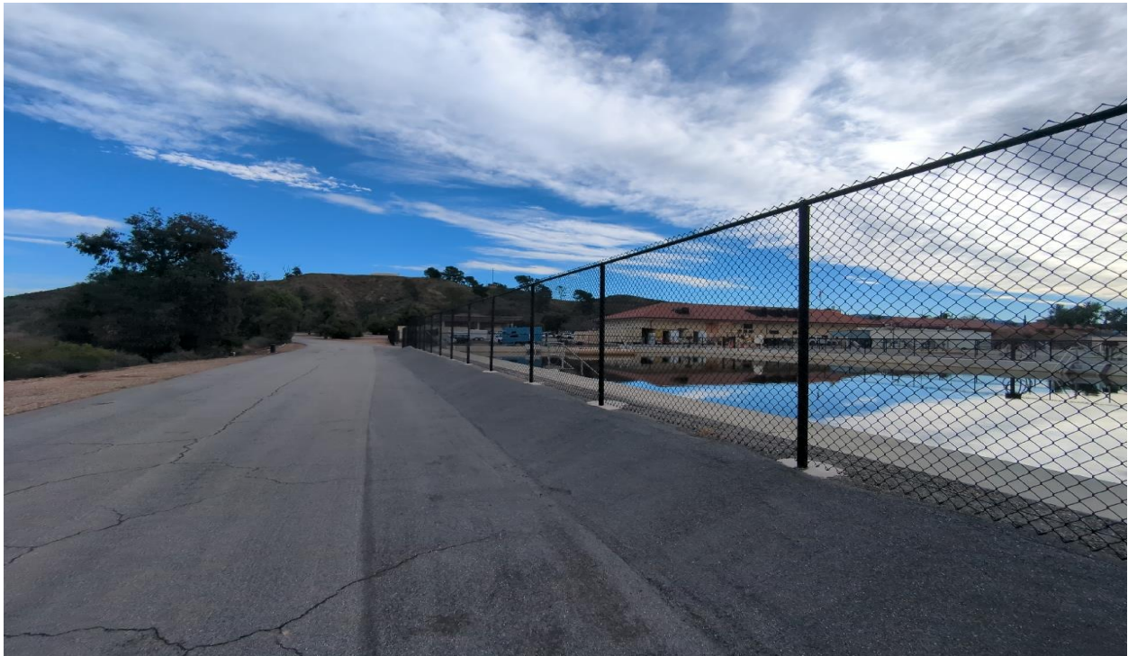
Photograph 14. View of existing water treatment facility associated with the RWTP, facing east.
