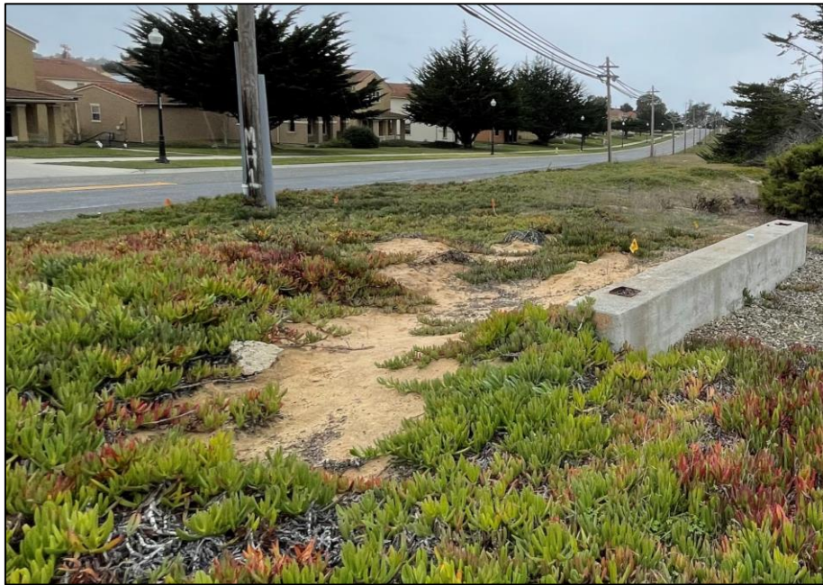
Photo 10: View of yellow flags for underground natural gas lines.
