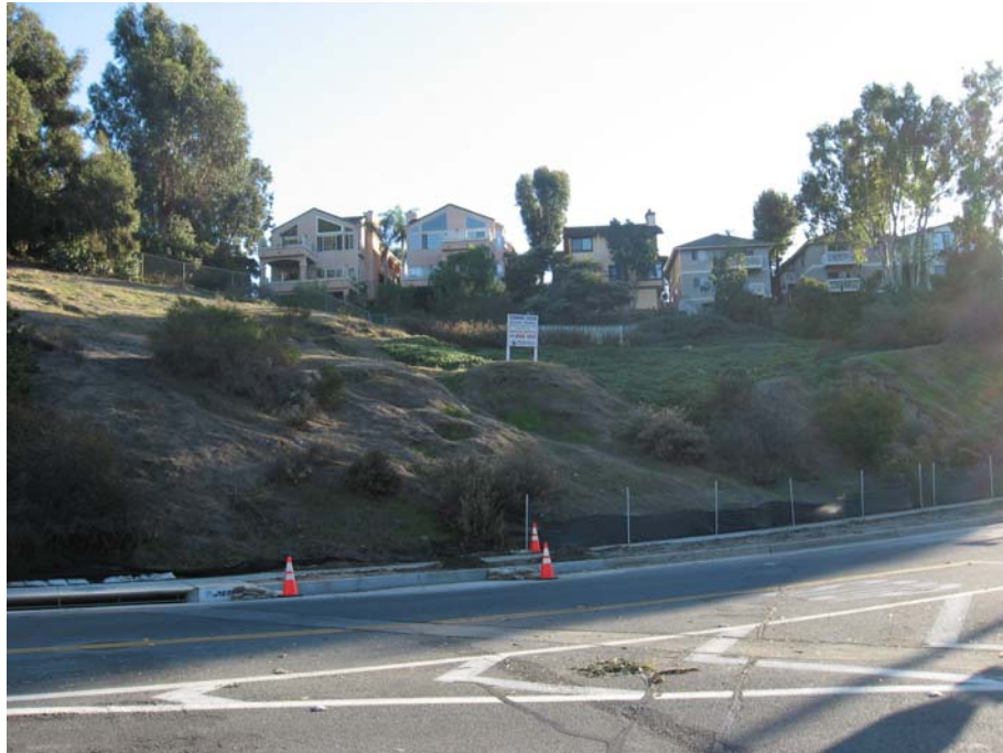
View of lots overlooking property near the west end. Notes piles of soil in the center of the slope associated with old erosion protection work.
