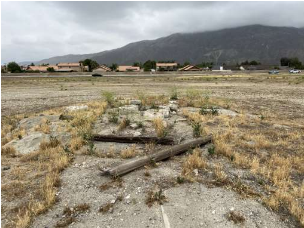
Photo 6: View of concrete rubble debris observed on central portion of the subject property.
