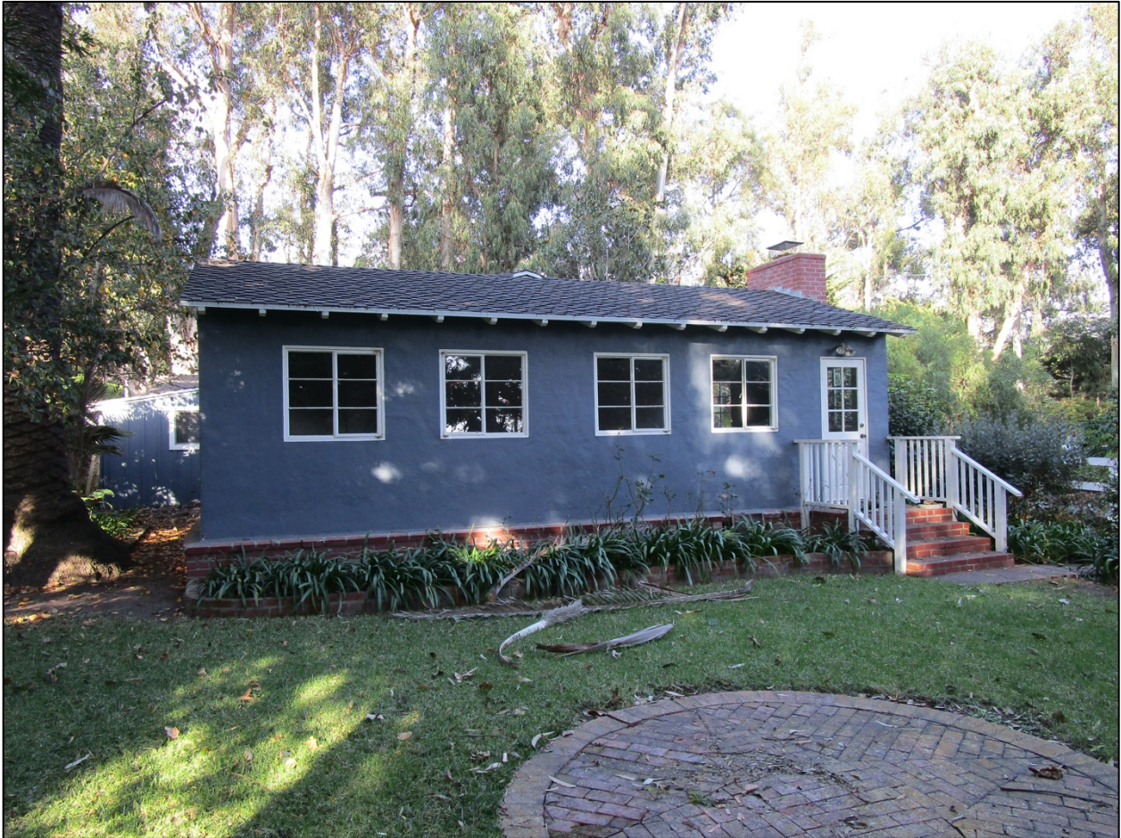
Caretaker's house, south elevation, looking north.
