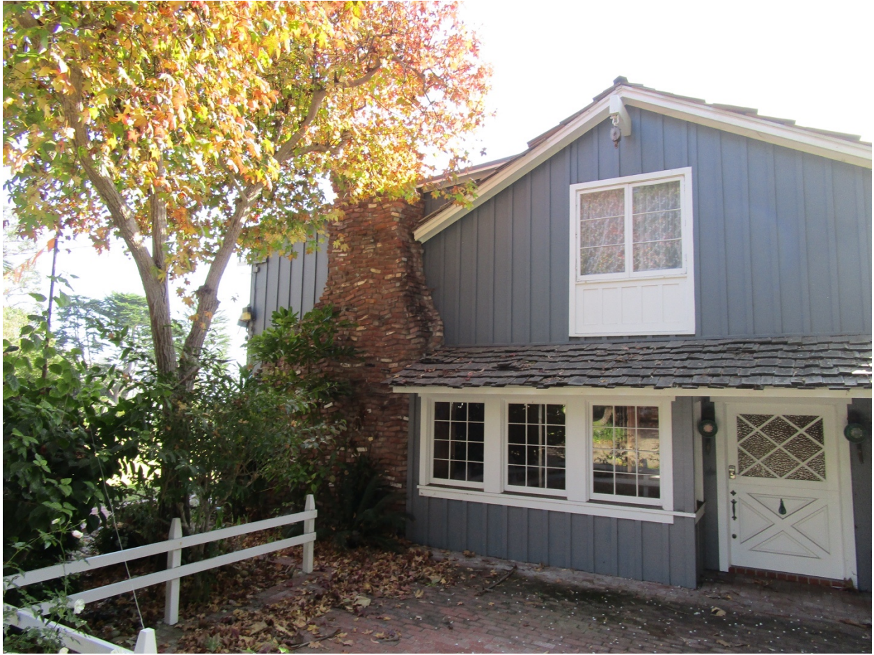
Main house, north elevation, looking southeast.
