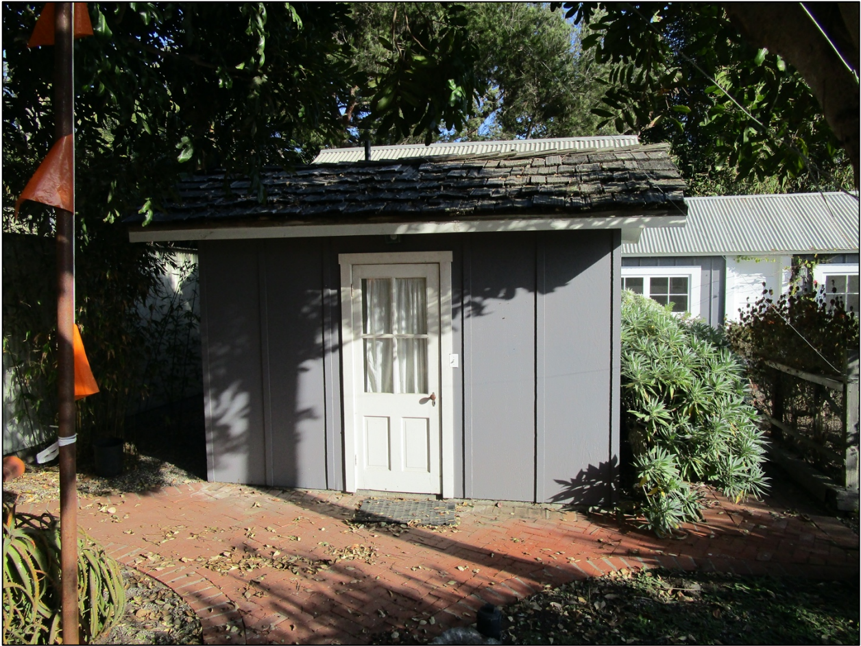
Bathroom shed, west elevation, looking east.
