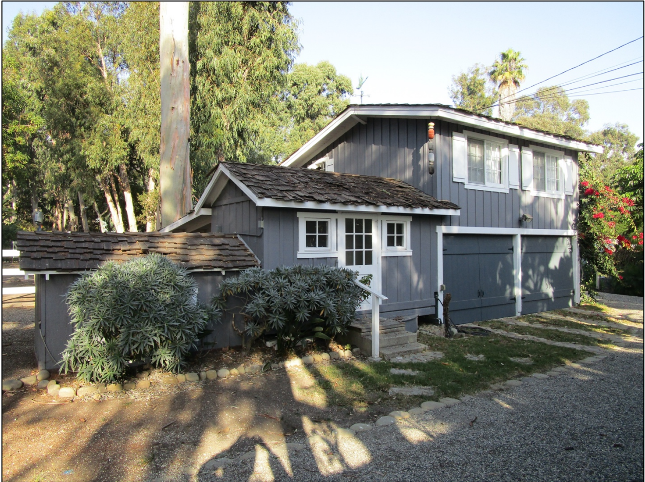
Office/Garage, south elevation, looking northeast.
