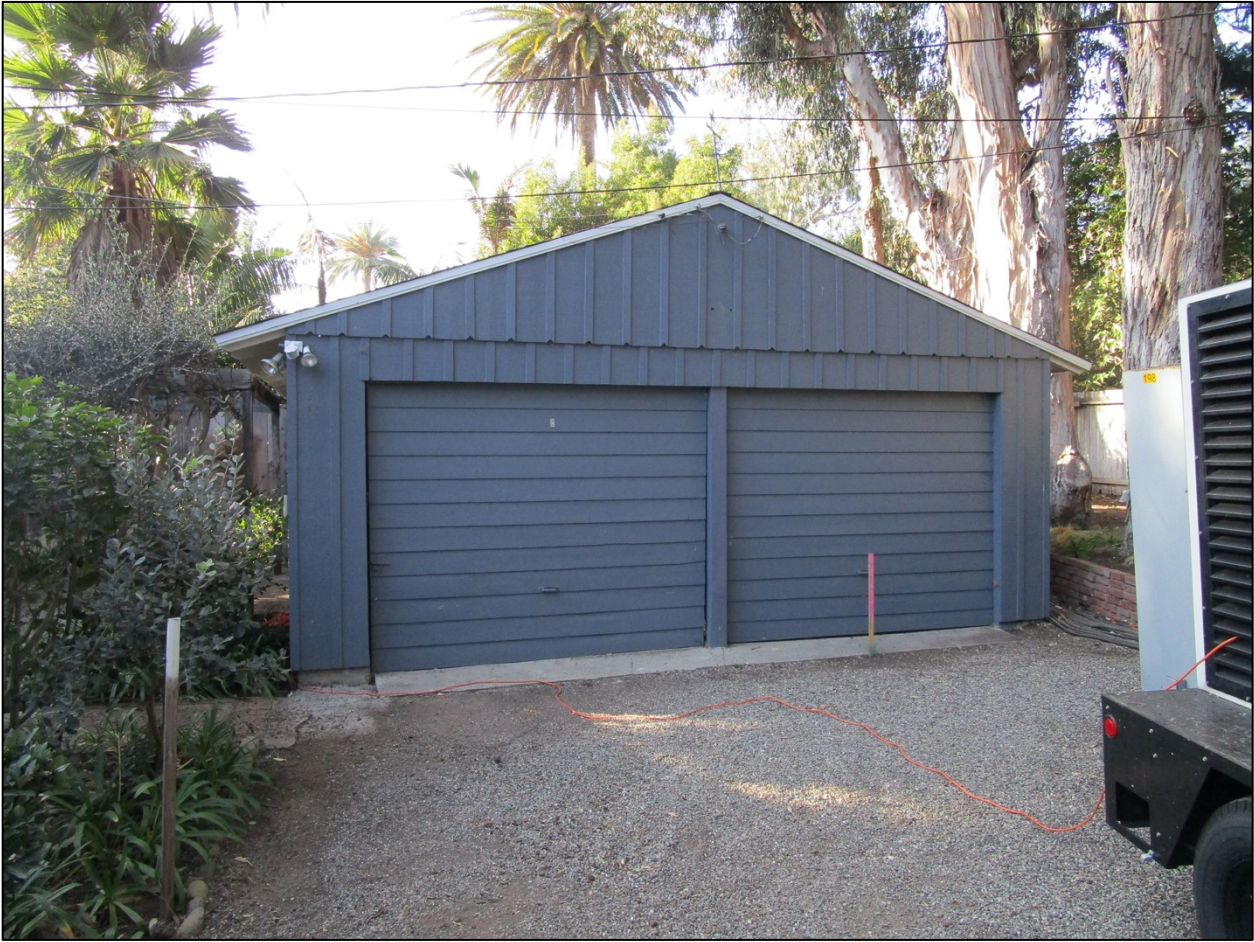
Garage, east elevation, looking west.
