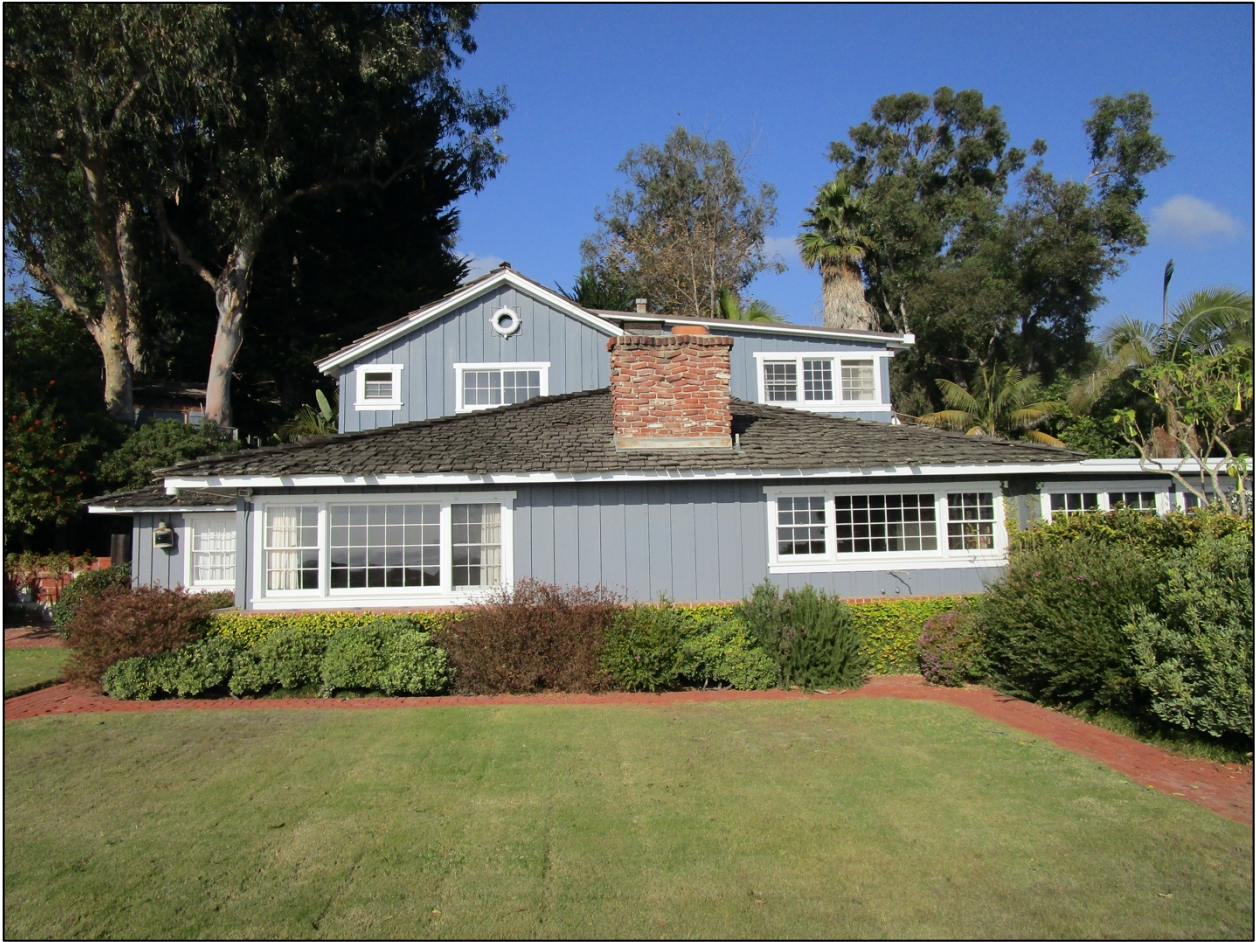
Main house, south elevation, looking north.
