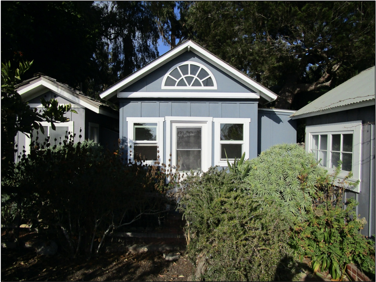
Change room, south elevation, looking north.
