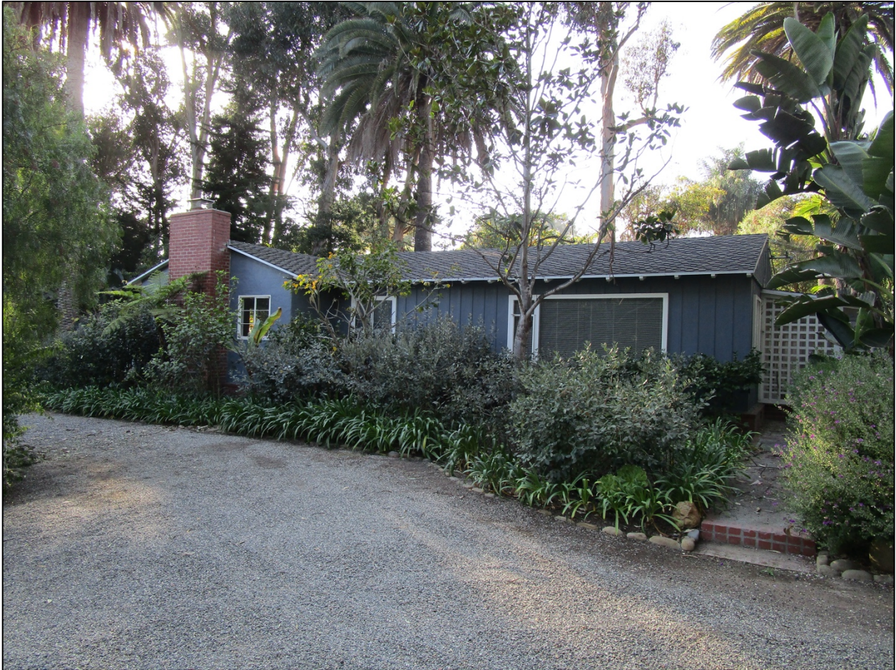
Caretaker's house, east elevation, looking west.
