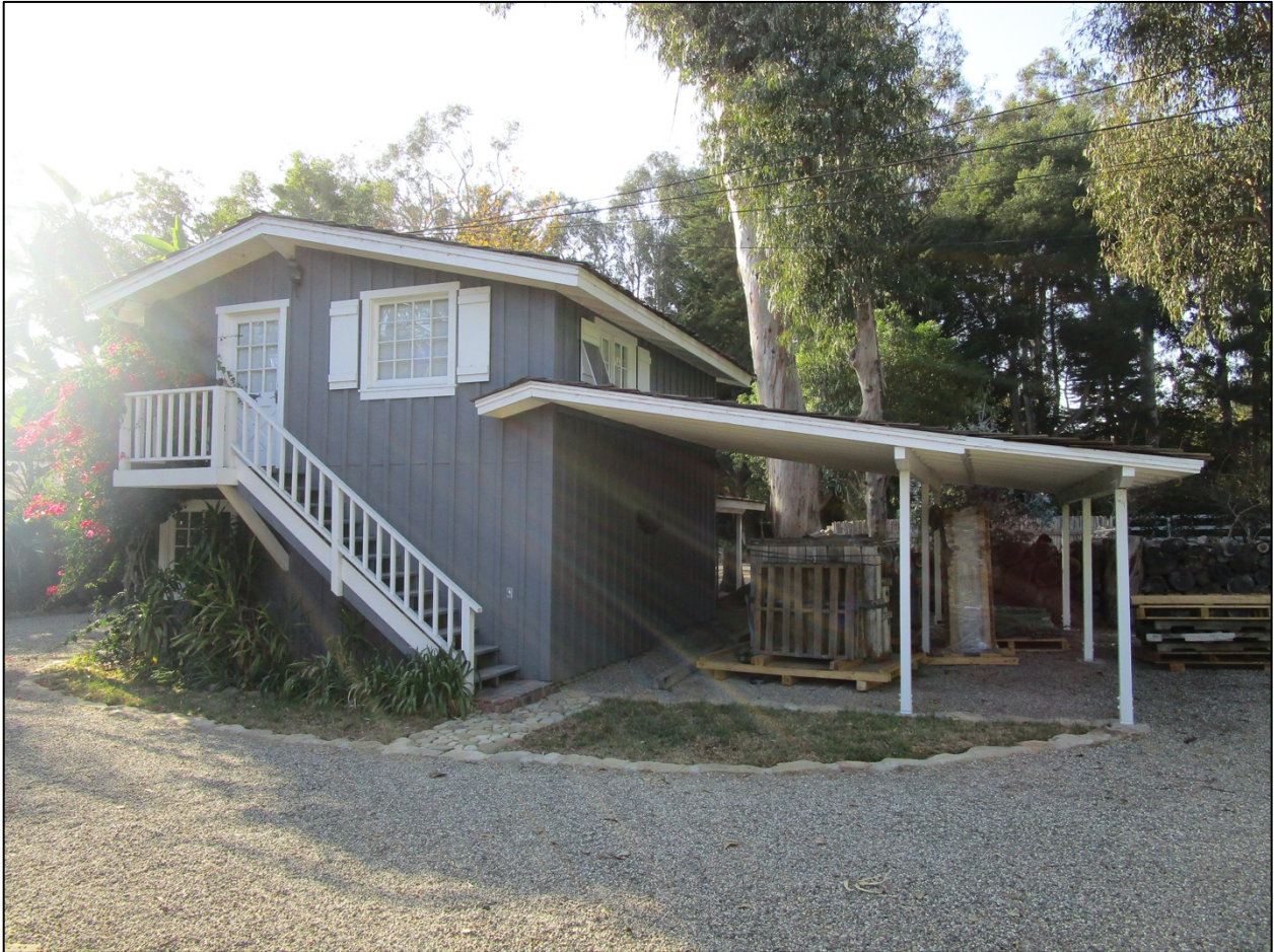
Office/Garage, east elevation, looking west.
