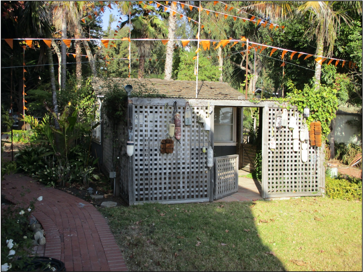
Small guest house, south elevation, looking north.
