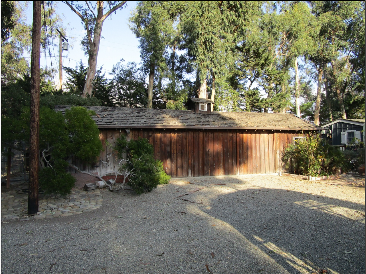
Garage/Workshop, south elevation, looking north.
