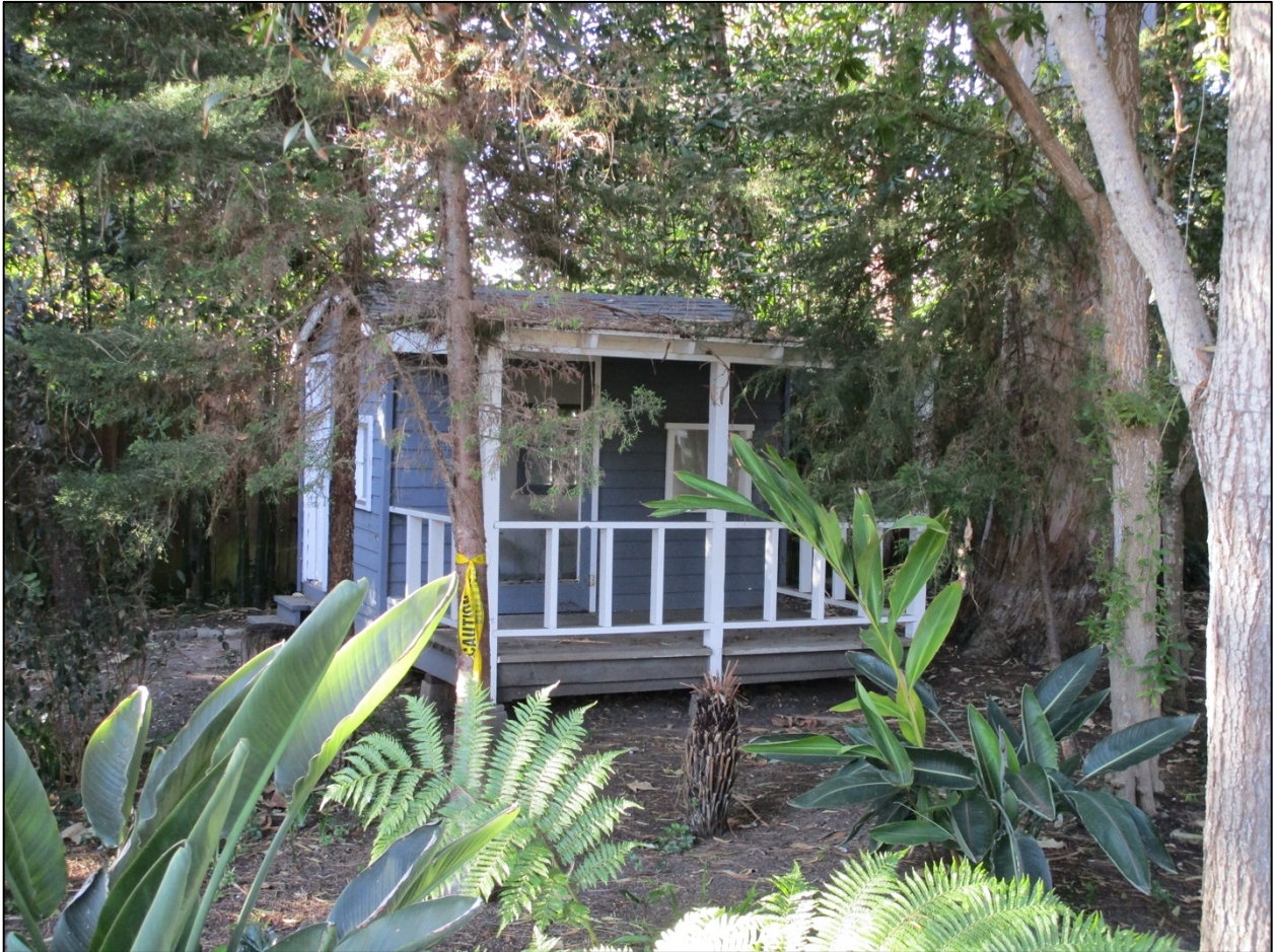
Playhouse, east elevation, looking west.
