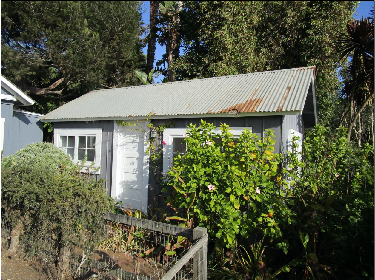
Bunk room, west elevation, looking northeast.
