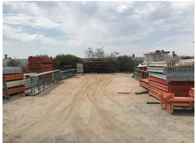
6. Additional scaffolding storage
