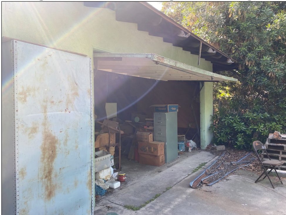
Figure 12. Exterior of Existing Attached Garage
