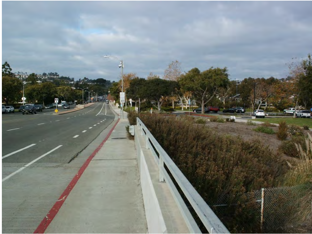
View of project area from north side of Stonehill Drive at San Juan Creek. Creekside Park on right. View to W. January 18, 2024.
