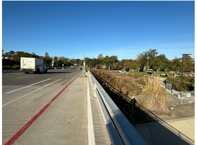
Photo 4: View looking west along Stonehill Drive at the eastern boundary of the project.
