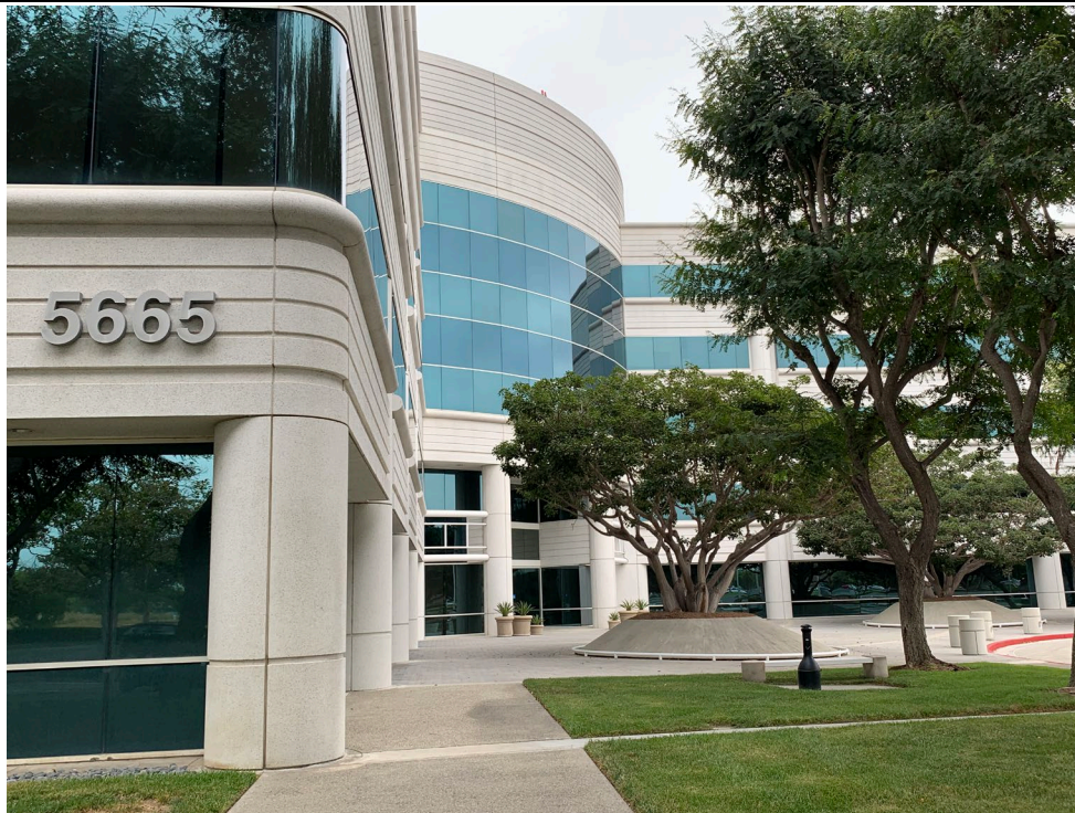
Photo #1 View of the 5665 Plaza Drive building exterior.
