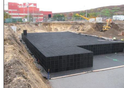
Underground detention tank Source: www.webtecgeos.com
