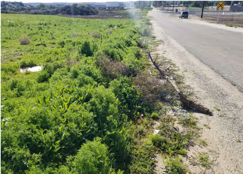
Photograph 1: View looking south along the eastern edge of the road improvement area.
