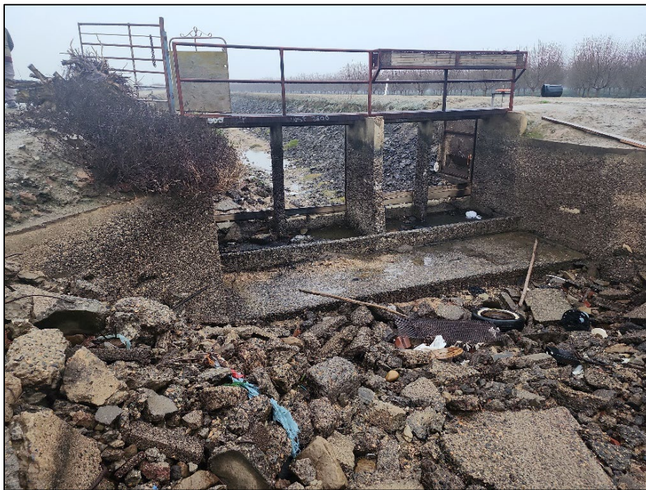
Figure 23. Check gate within Houghton Canal segment, facing slightly southeast.
