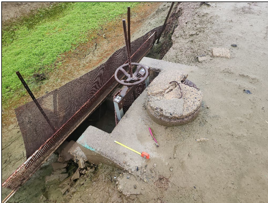
Figure 26. Turnout 23, facing northwest.
