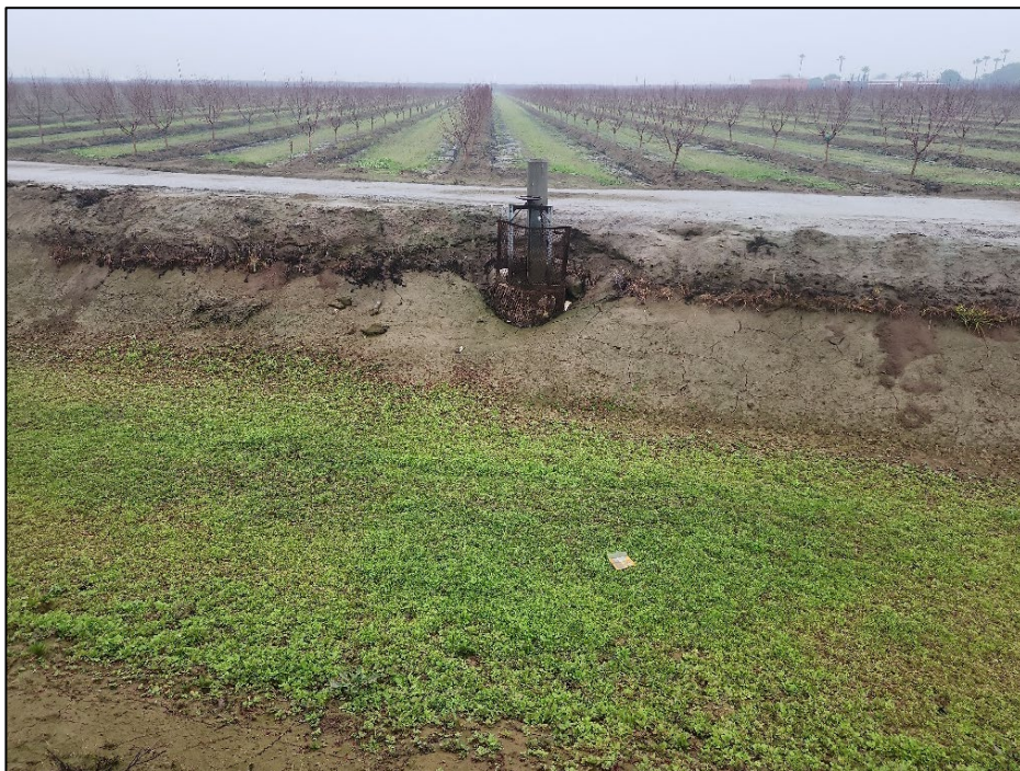
Figure 28. Turnout, facing west.
