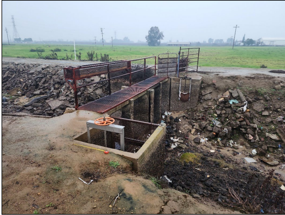
Figure 22. Check gate within Houghton Canal segment, facing north.
