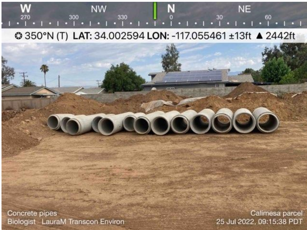
Photo 2. Depicts the materials staged on the graded project site.
