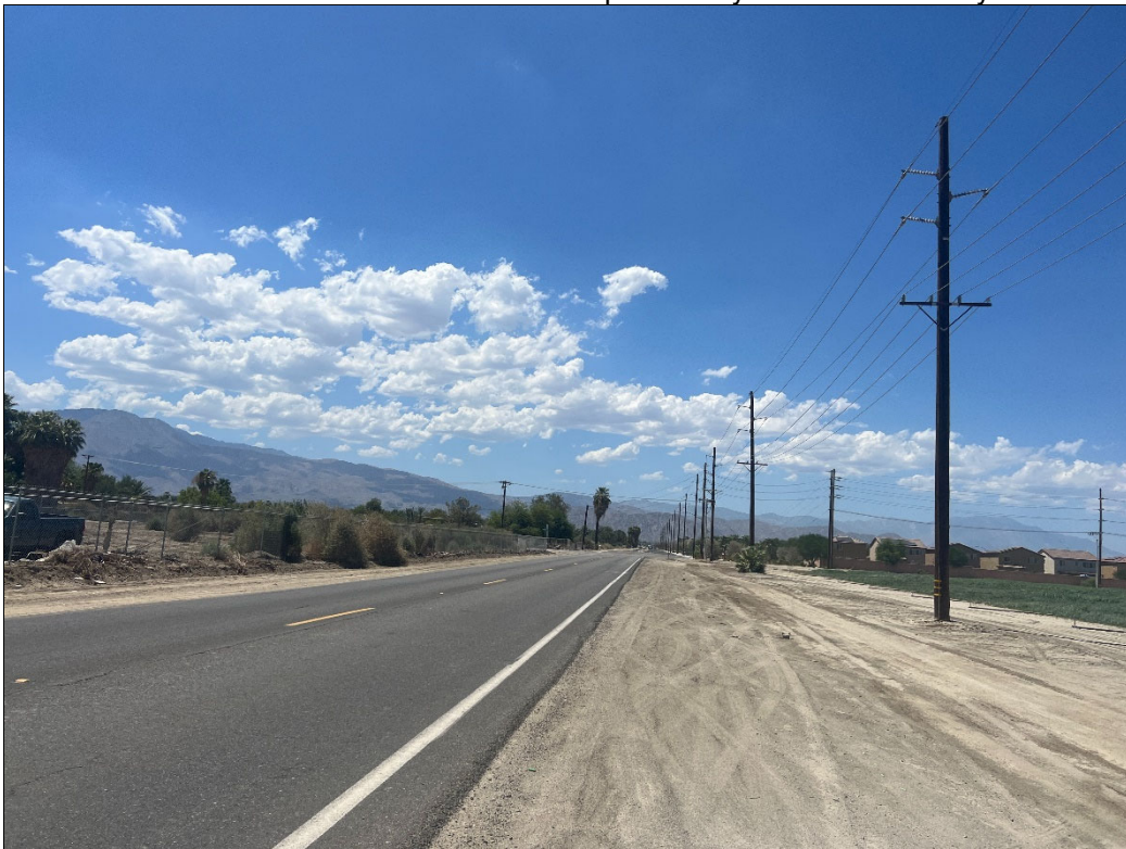
Photo 10. Project route along Ave. 54 east of Shady Lane. Note residential development in background.
