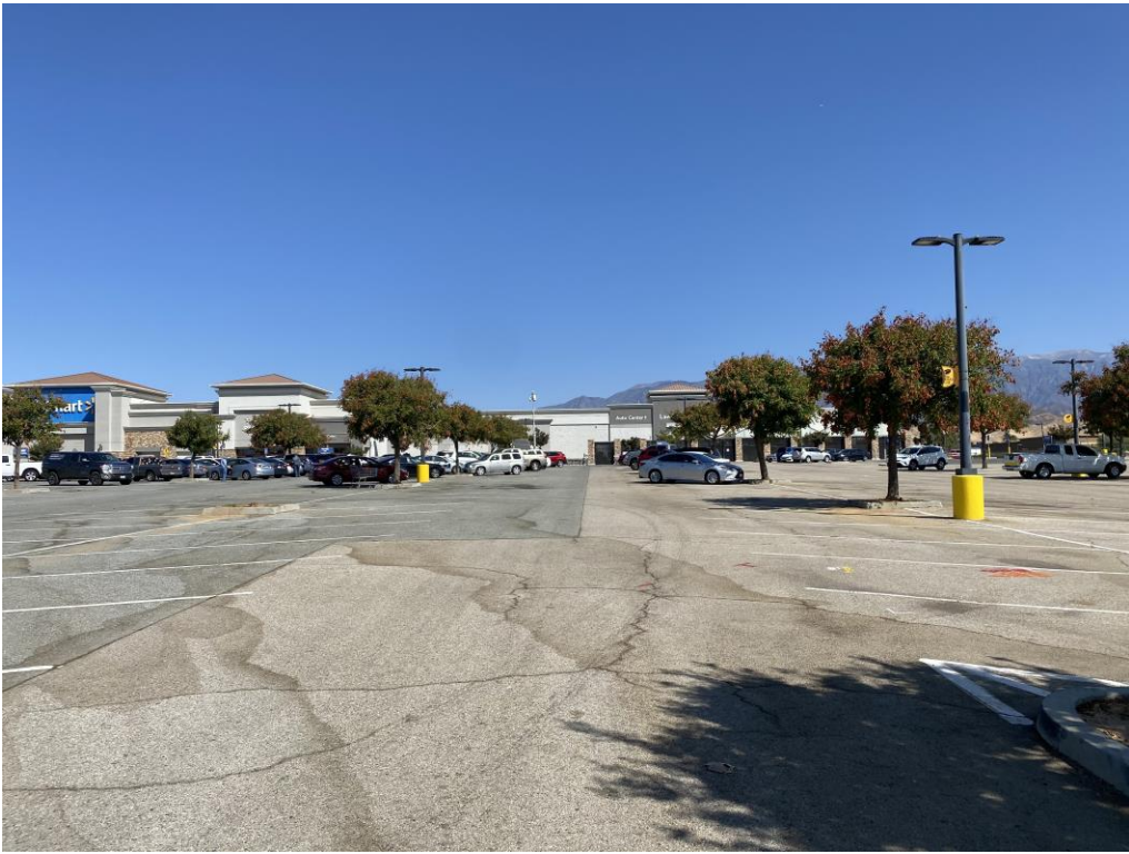
Photo 5: View of subject property from the southwest corner facing north.
