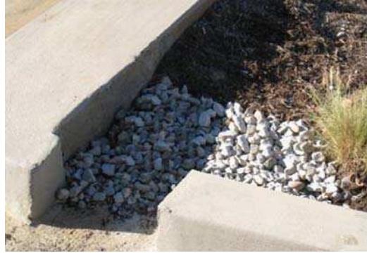
Figure 2: Curb Cut located in a Bioretention Facility
