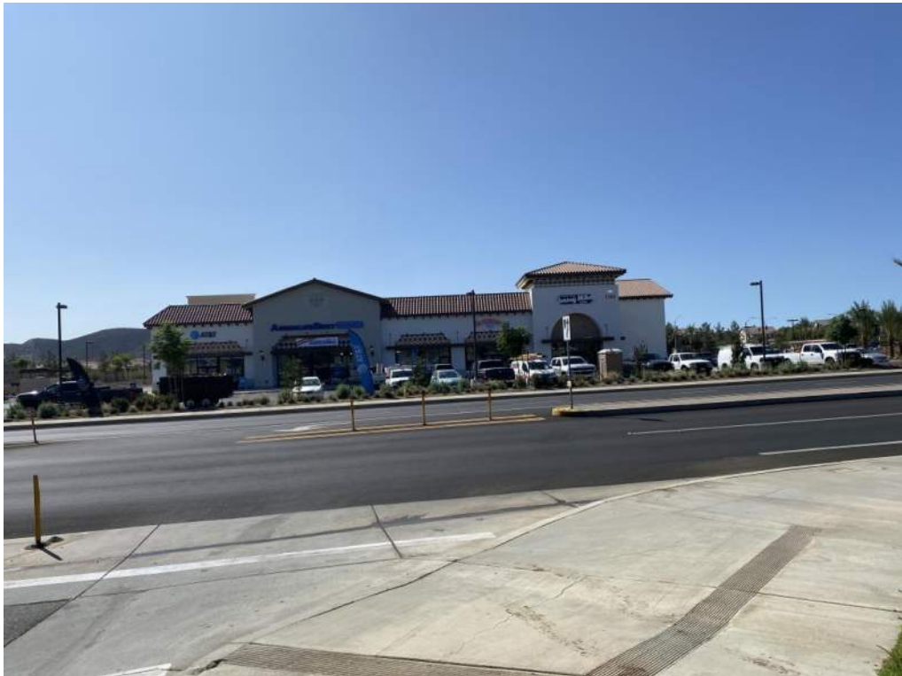
Photo 10: View of adjoining property to the adjoining property to the south.
