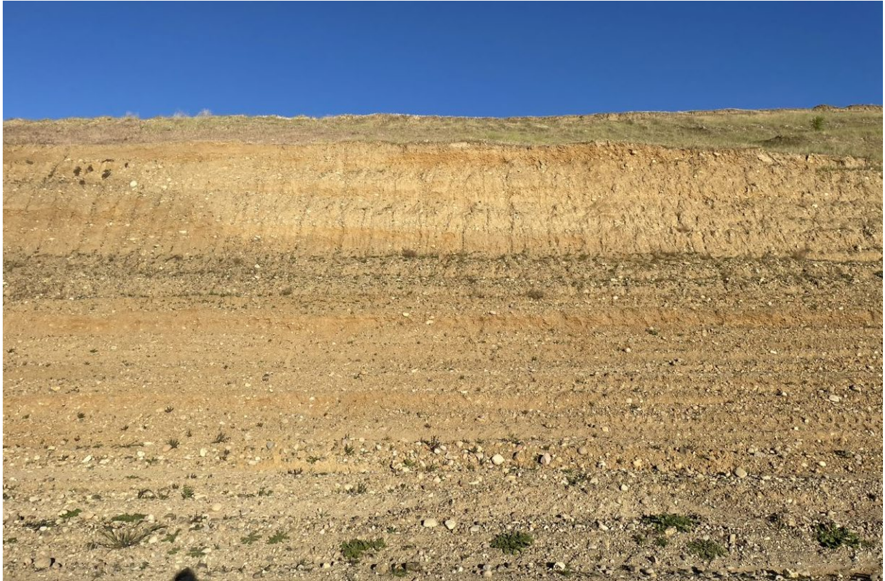
Photo 3: Eastern cutslope in Pit 4, looking east (taken 03-07-2022)
