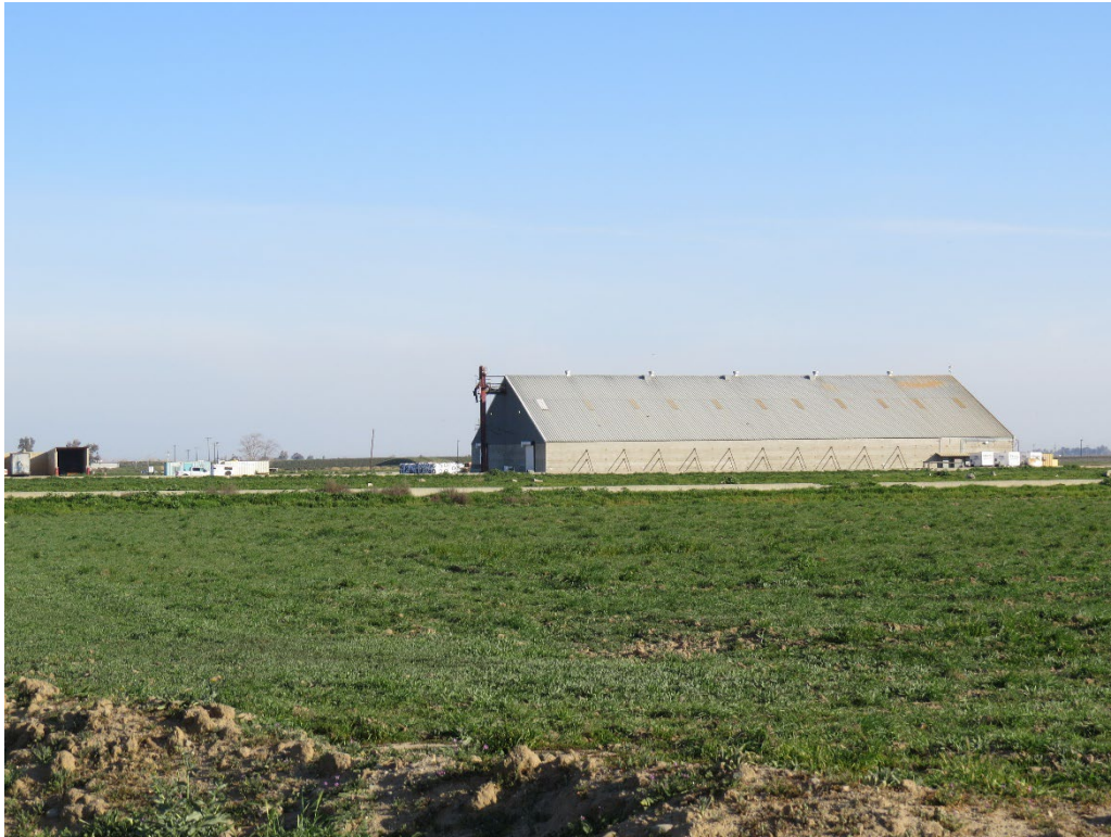
Photograph 5: Looking at the existing structure in the middle of the Turner site.
