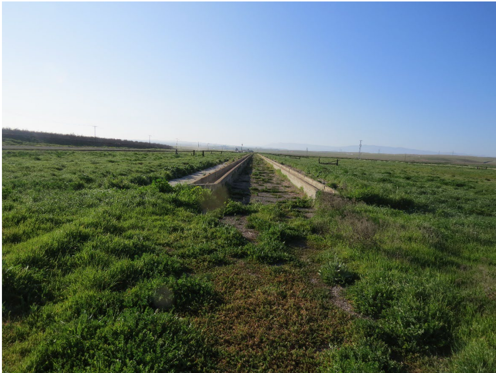
Photograph 4: Looking south at the western half of the Turner site.
