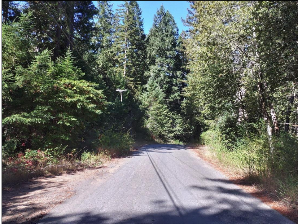
Photo A-5. Fort Ross Road, facing west. Habitat consists of redwood forest along left shoulder and riparian habitat along right shoulder. Photo taken 10/3/2023.
