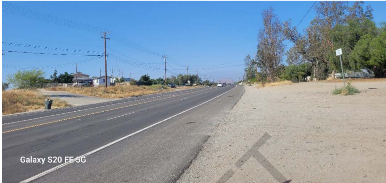
Photo No. 3: Hwy 74, view towards northeast.
