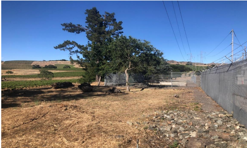
Photo 6. Facing south from the Northwest corner of the Tulucay PG&E Substation where expansion is proposed.
