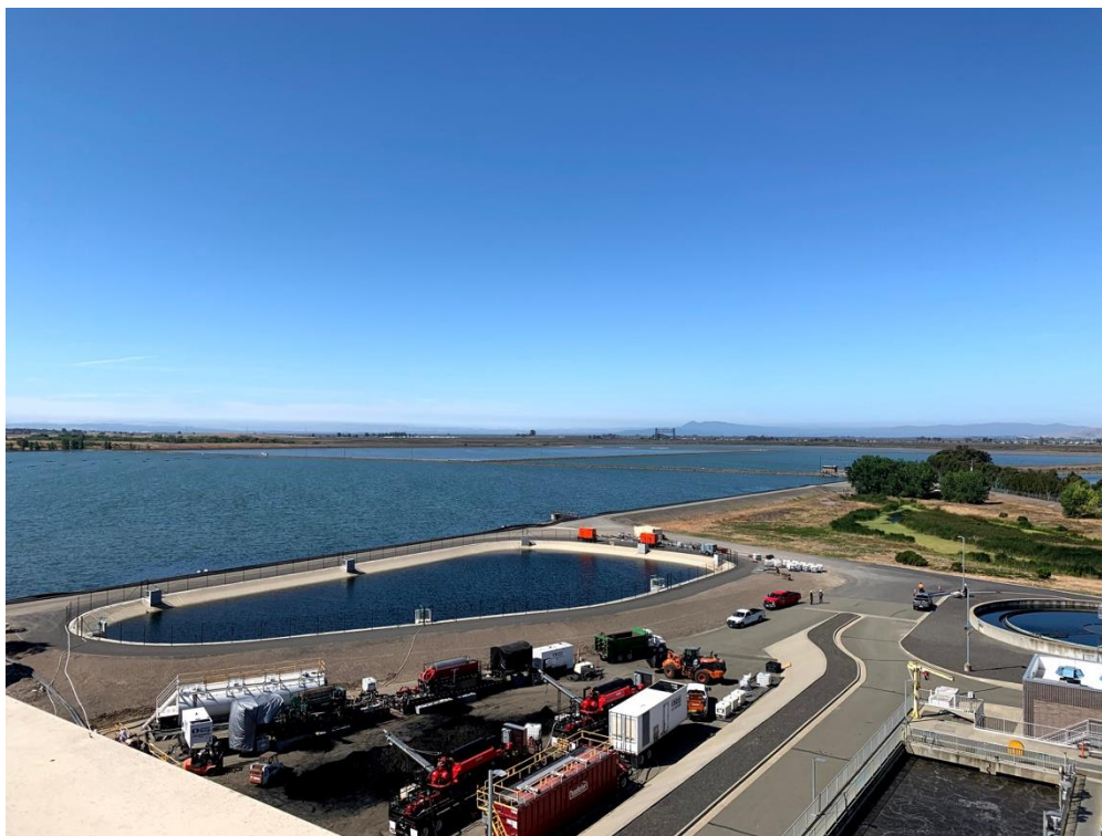
Photo 1. Project Study Area facing southwest toward ponds 3 and 4.
