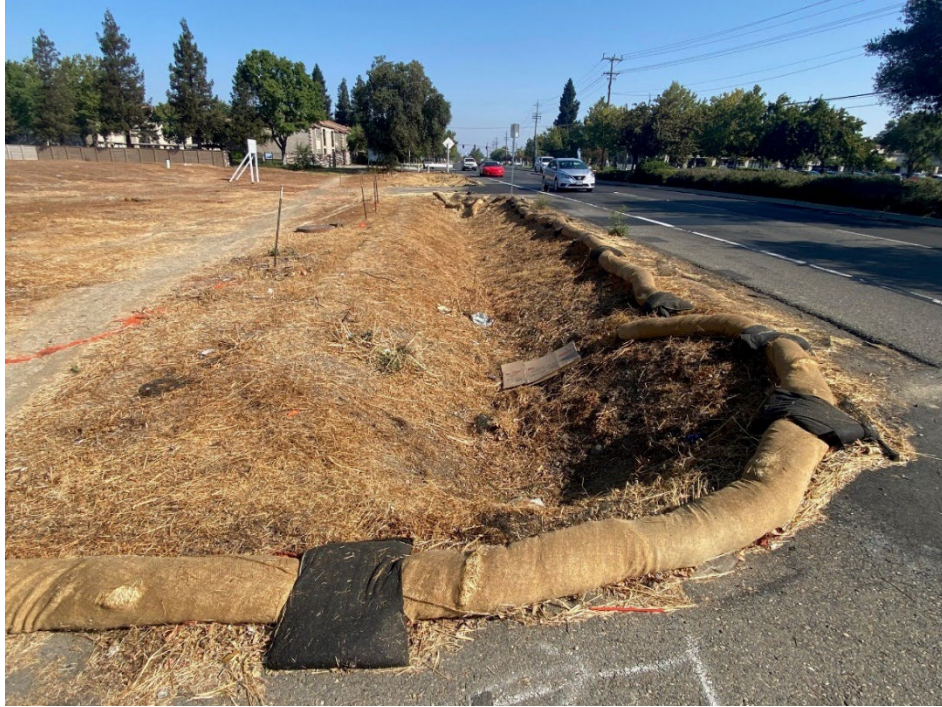
Photo 11: Ditch and view of southern adjunct trail alignment in Segment 1; facing north.
