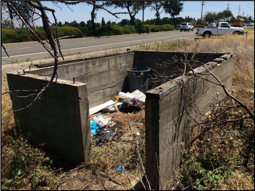
Figure 8. P-34-005386/CA-SAC-001278H, F-001 concrete board-formed structure, view southeast
