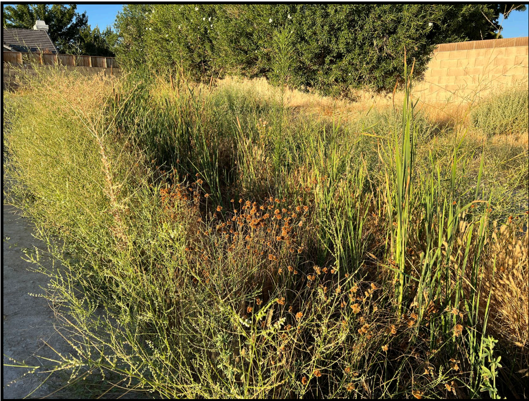
Storm drain, oriented north-south inside western boundary. Top photograph is north side looking south. Bottom photograph is view of the last southern 100 feet of the storm drain.
