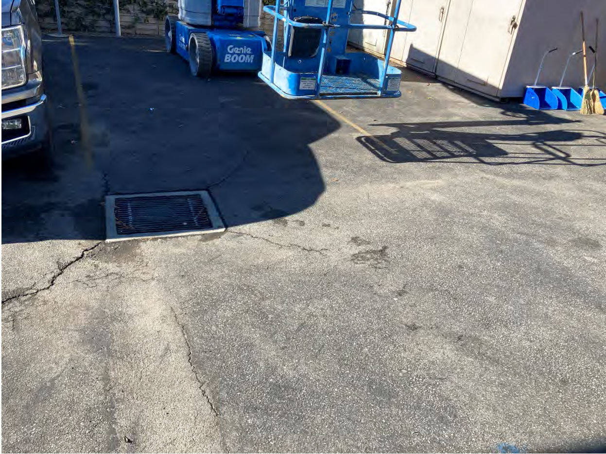
Floor drain located in center of maintenance yard area.
