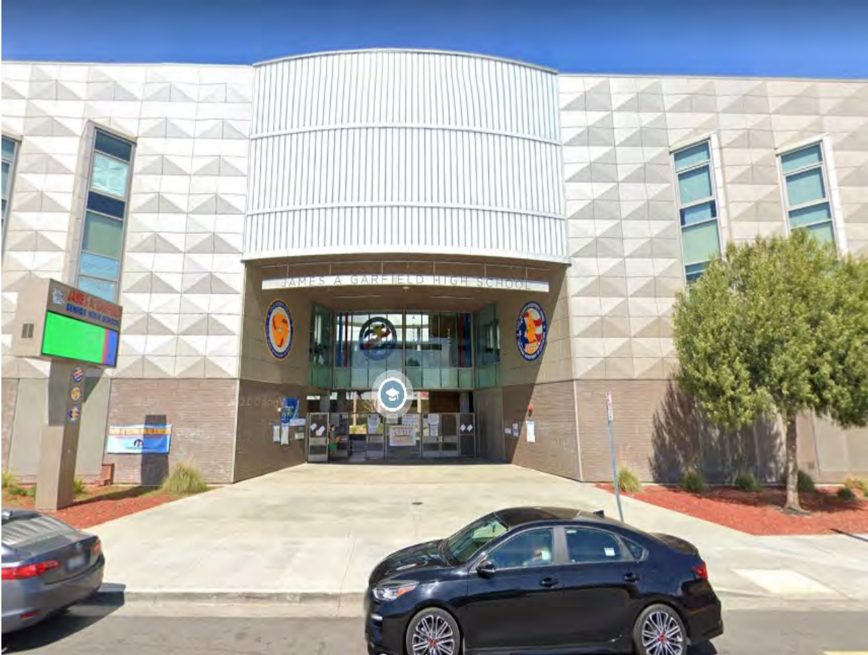
James A. Garfield south entrance facing north.
