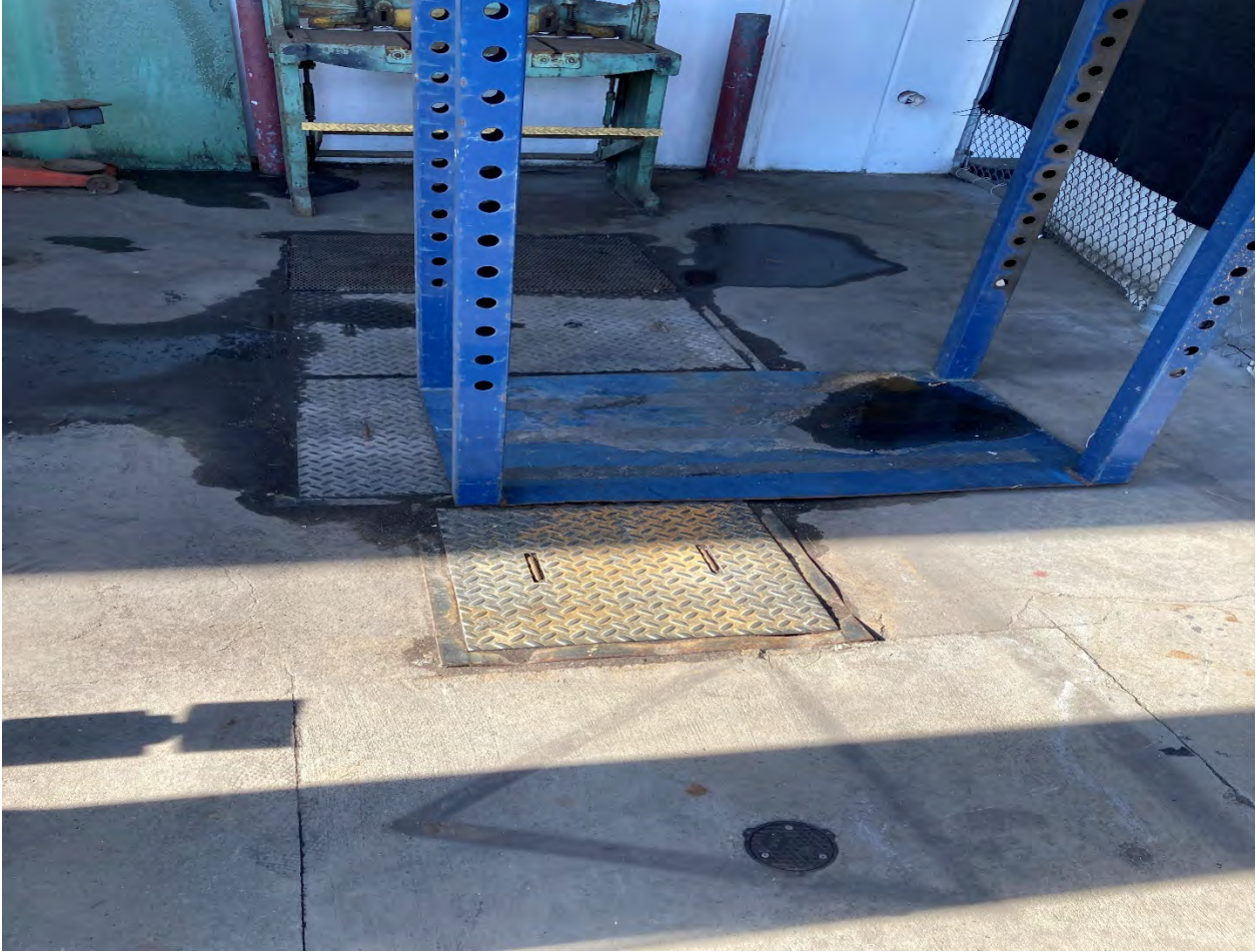
Northeast corner of Auto shop yard. 3-stage clarifier observed.
