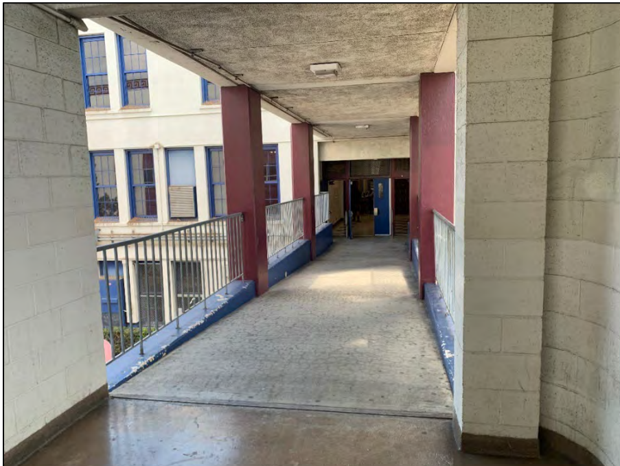
Figure 10. West façade of the Science Building, showing the arcades connecting to the Library/Classroom Building. View to the southeast. The arcades will be demolished along with the Library/Classroom Building in the foreground.
