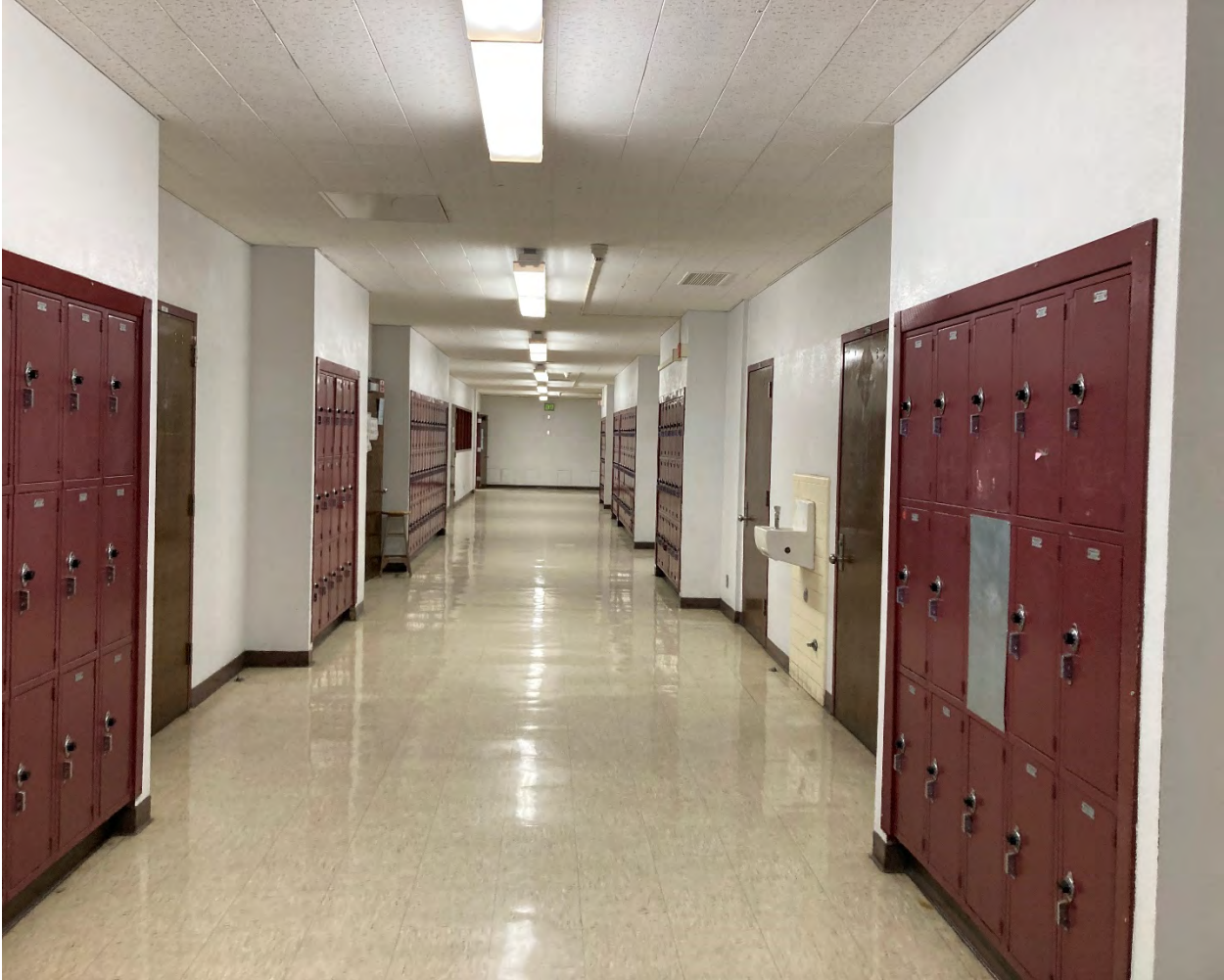
Building 200 interior main corridors.
