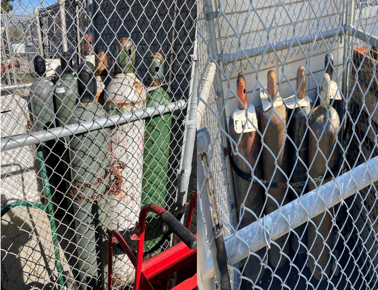
East and northeast ends of Auto shop yard. Full bottles of compressed air used for shop processes stored in cages.
