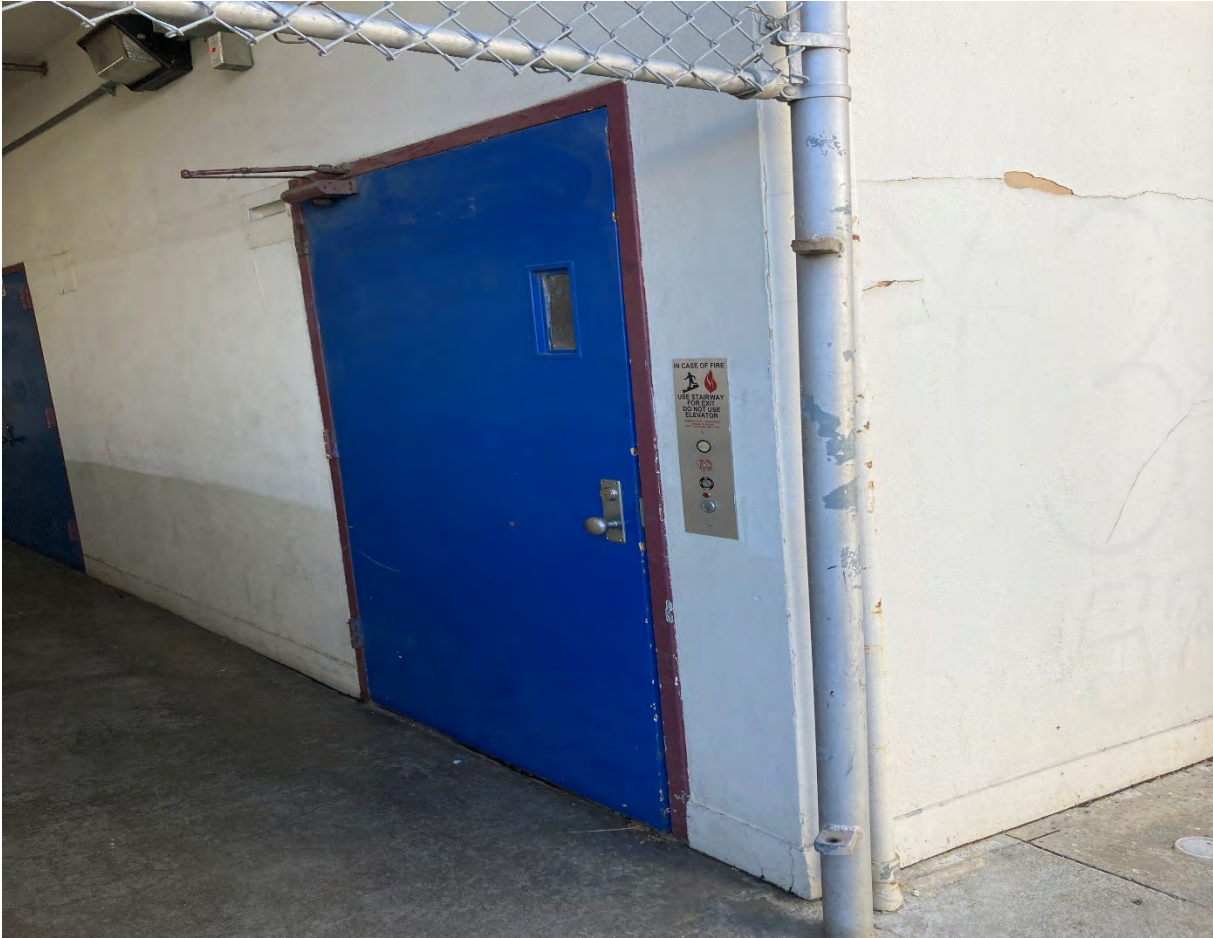
Out of use freight elevator located on exterior of building 500.
