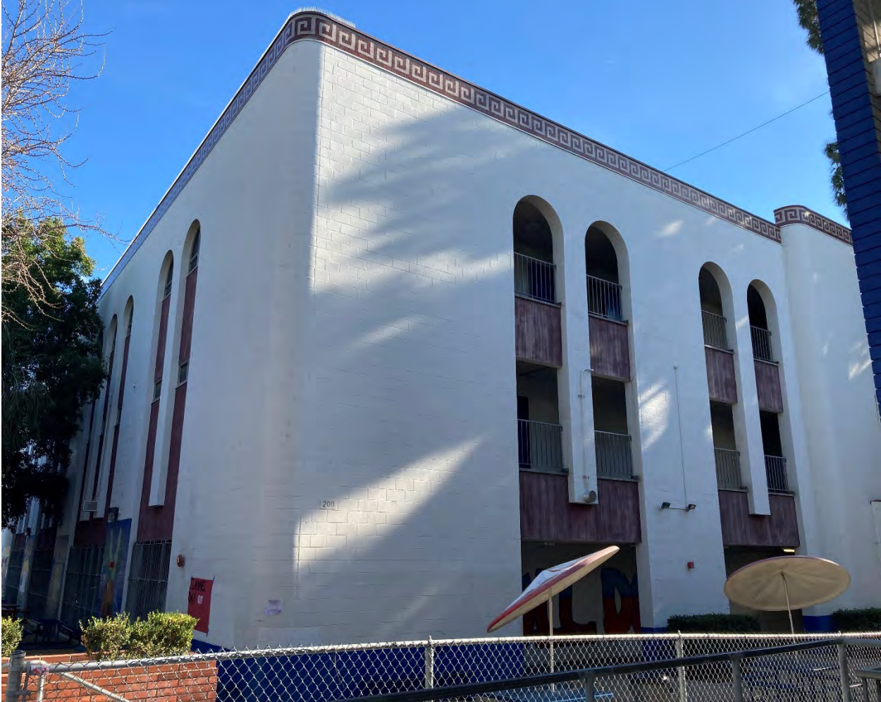
Southeast corner of building 200.
