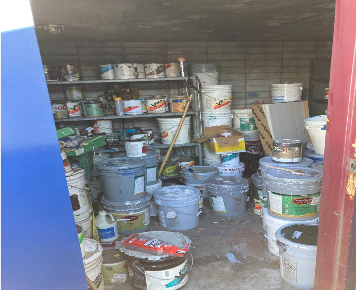
Paint storage room located at west end of campus in maintenance yard.
