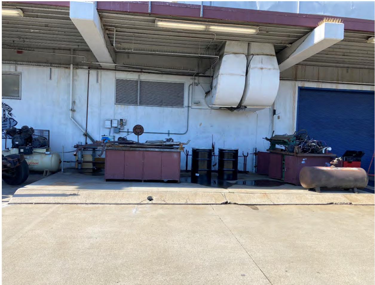
Auto shop yard located on the east end of campus. Garfield High School Wellness Center adjacent from the auto yard. East end of yard facing north. Two waste drums (used oil and coolant) are stored in the yard on an elevated concrete slab as a secondary containment. Two empty storage tanks for gas are also stored near the area.
