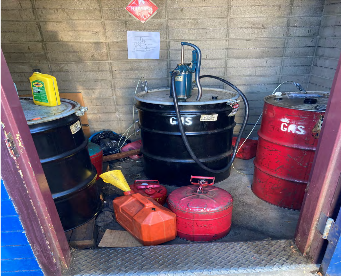
Fuel storage room with secondary containment within located on west end of campus in maintenance yard adjacent to maintenance offices.
