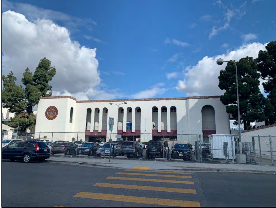
Figure 11. South façade of the Library/Classroom Building, view to the north, showing mosaic medallion.
