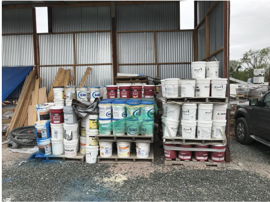
Photograph 21: Paint storage on WM O'Neill portion of the Site.
