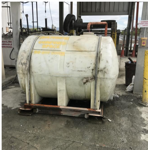
Photograph 10: Water aboveground storage tank on Pick-N-Pull portion of the Site.
