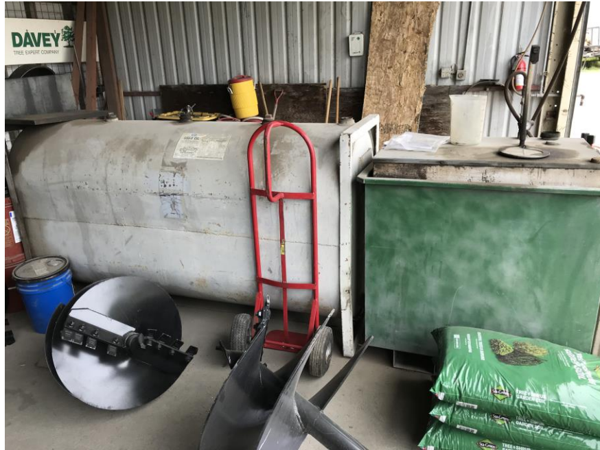
Photograph 19: Unused waste-oil aboveground storage tank and parts washer in storage warehouse on Davey Tree portion of the Site.
