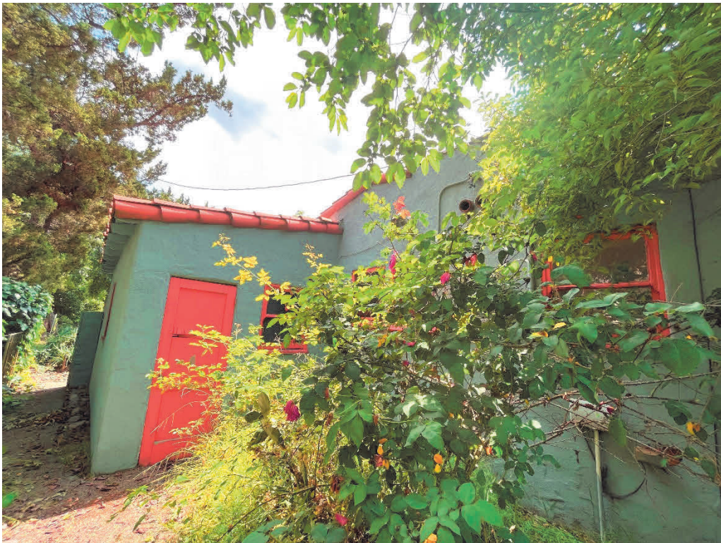
Figure 15. Detail of eastern façade, view toward south.
