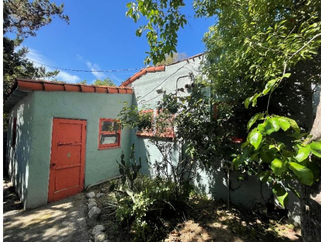
Figure 8A. Eastern Façade (view southwest) SOURCE: Sapphos Environmental, Inc., 2022
