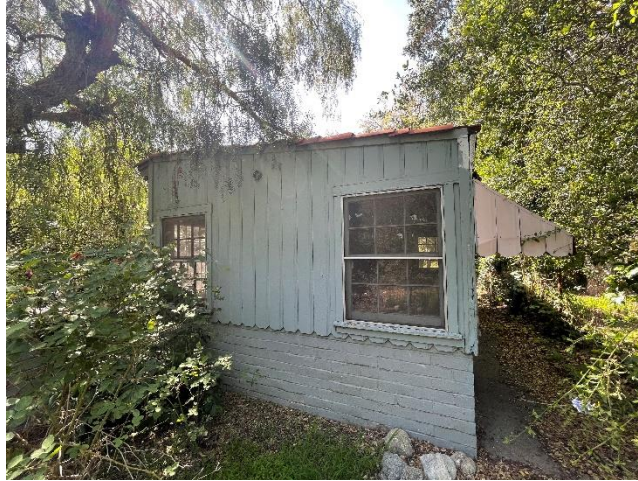
Figure 7C. Northern Façade (rumpus room addition; view south) SOURCE: Sapphos Environmental, Inc., 2022
