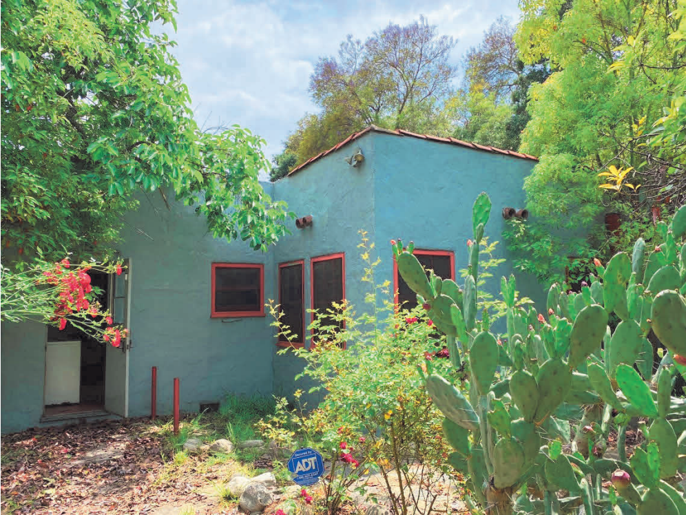
Figure 12. Detail of rear façade, view toward south.
