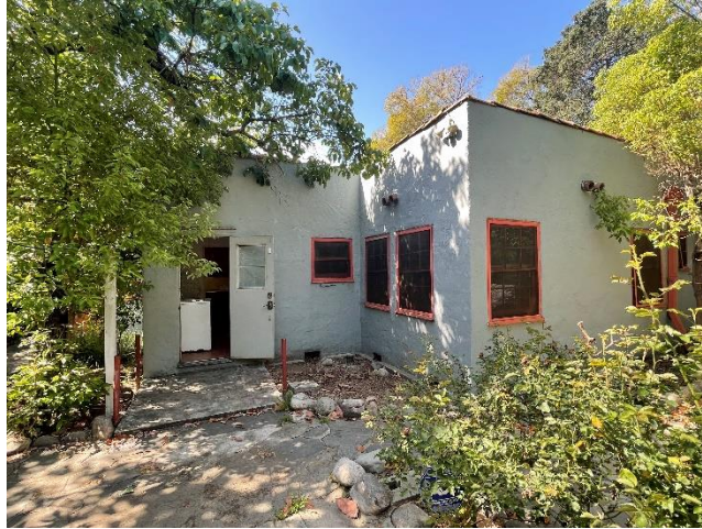
Figure 7A. Northern Façade (view southwest) SOURCE: Sapphos Environmental, Inc., 2022
