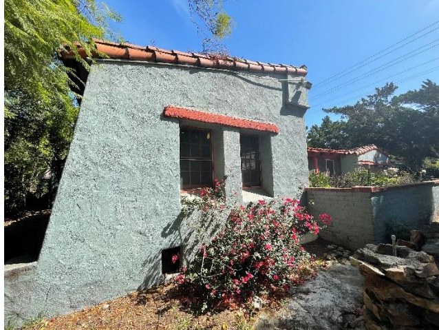
Figure 6G. Primary Façade (view north) SOURCE: Sapphos Environmental, Inc., 2022
