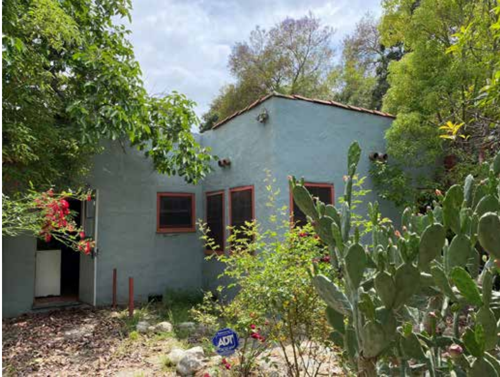
Figure 9. Detail of rear façade, view toward south.
