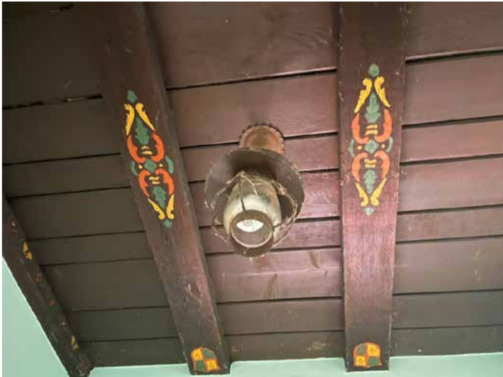
Figure 14. Detail of painted patterns and crests on entrance hall ceiling.
