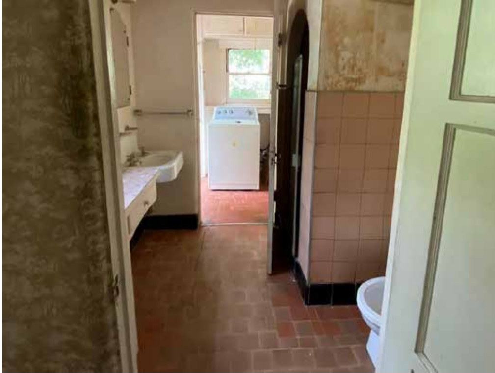
Figure 21. Rear bathroom, view toward east.
