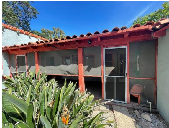
Screened Porch Detail (view north)
