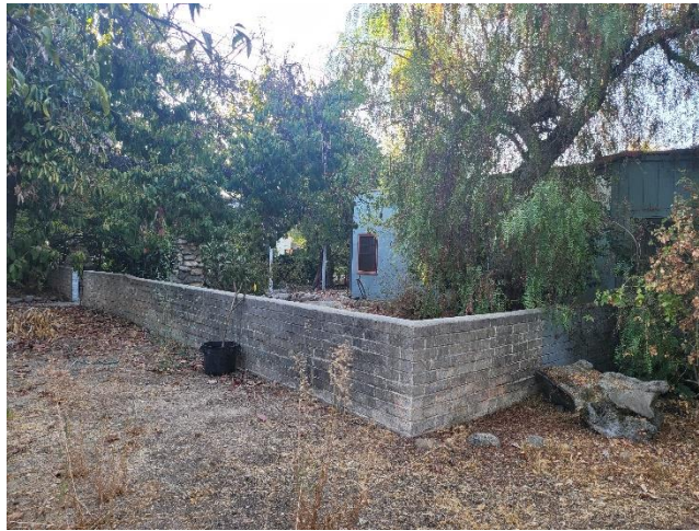
Figure 7D. Northern Façade (block wall; view southeast) SOURCE: Sapphos Environmental, Inc., 2022
