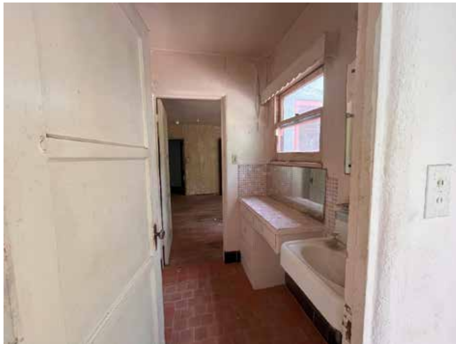
Figure 20. Rear bathroom, view toward west.
