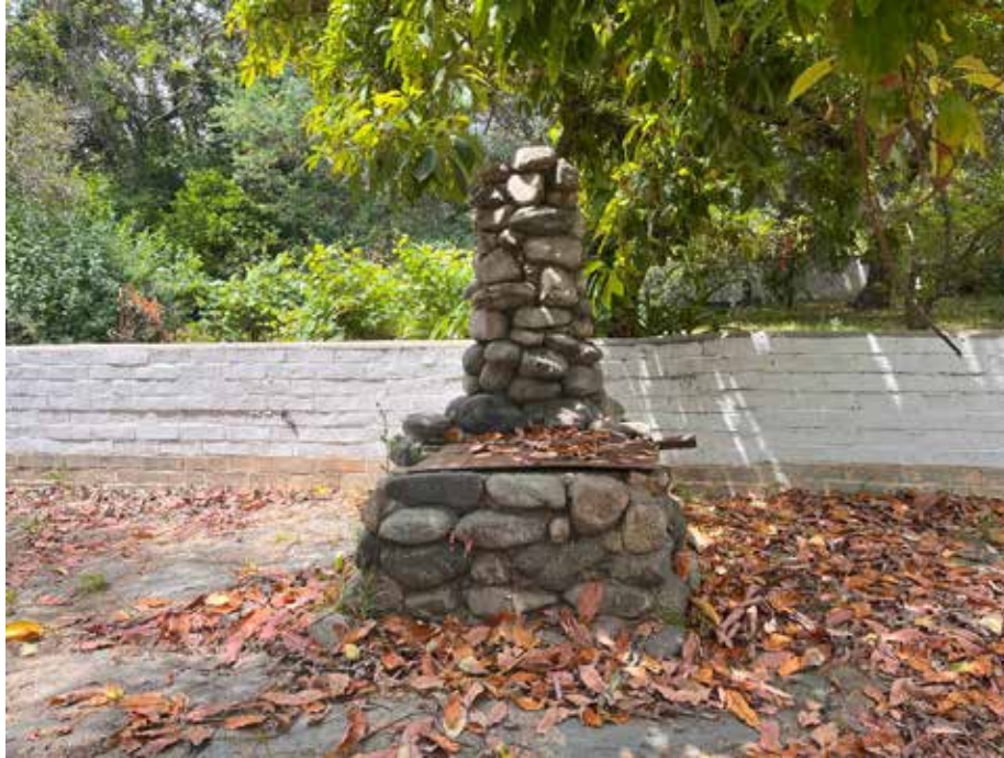
Figure 11. Detail of exterior stone fireplace. View toward north.
