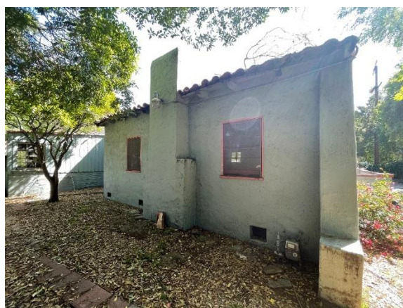
Western Façade (view northeast)
