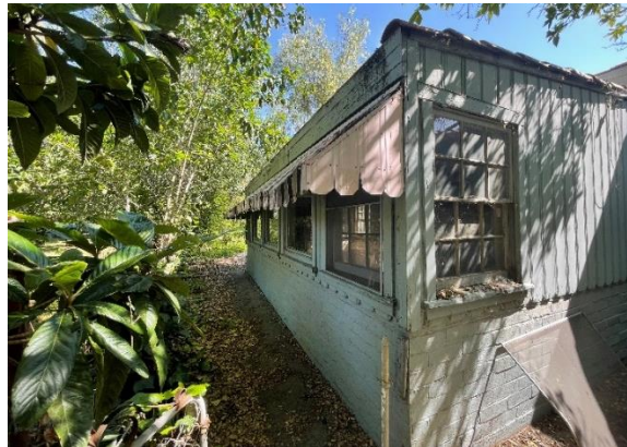
Western Façade (rumpus room addition; view northeast)
