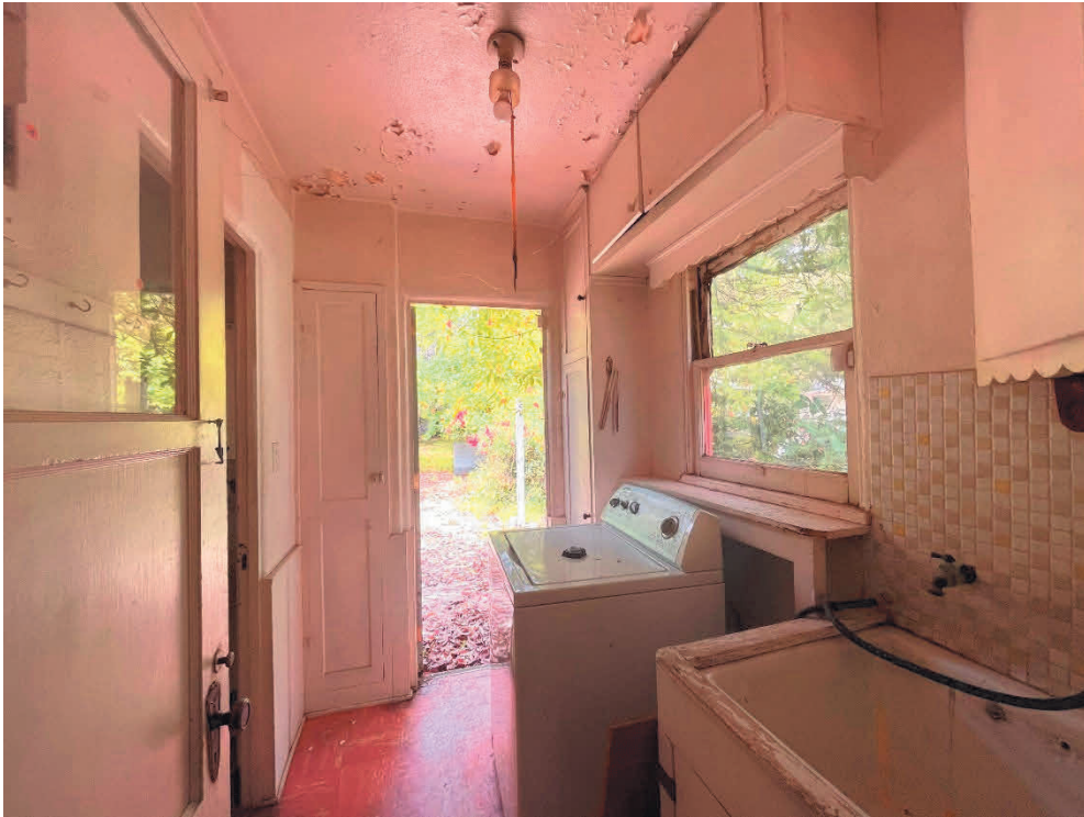
Figure 22. Laundry room and rear exit, view toward north.
