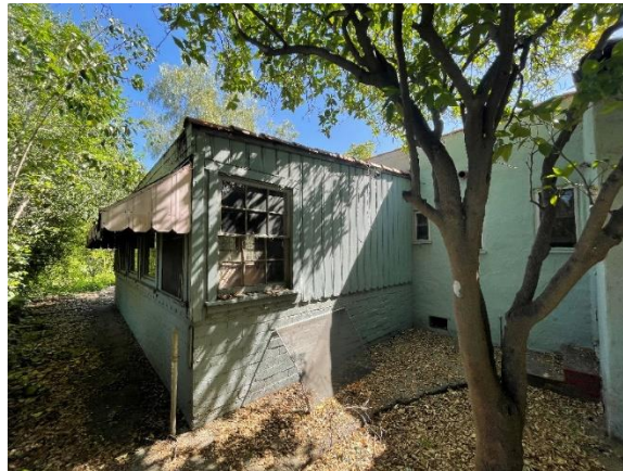
Western Façade (view northeast)
