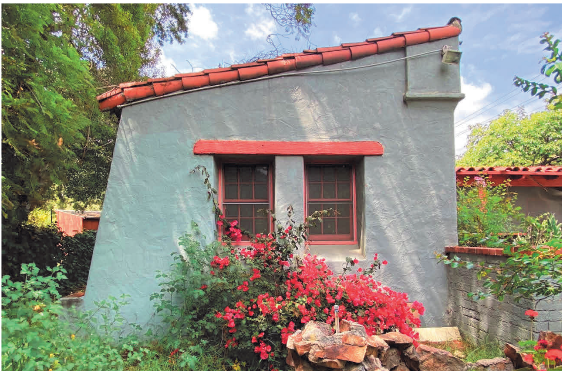
Figure 5. Detail of shed roof section, view toward north.
