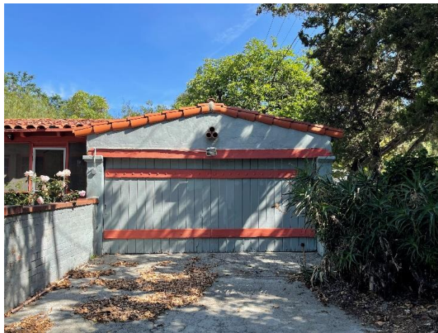
Figure 6H. Primary Façade (view north) SOURCE: Sapphos Environmental, Inc., 2022
