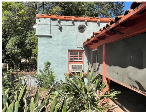
Primary Façade (view west)
