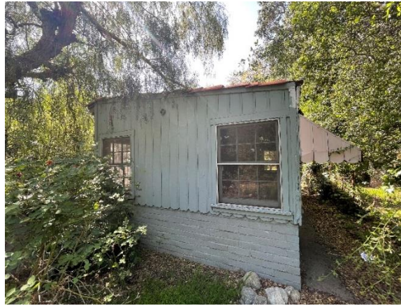
Northern Façade (rumpus room addition; view south)
