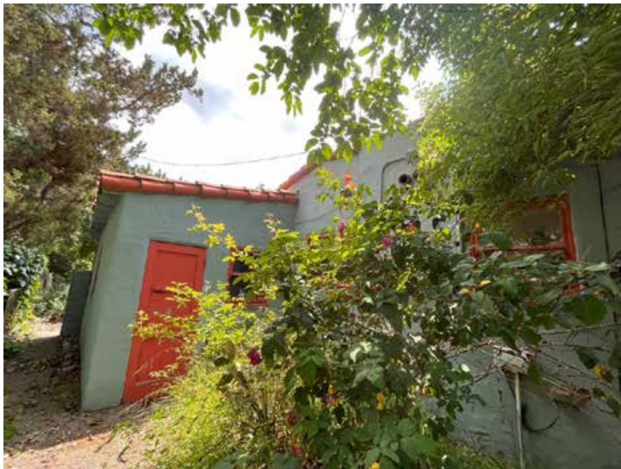
Figure 12. Detail of eastern façade, view toward south.
