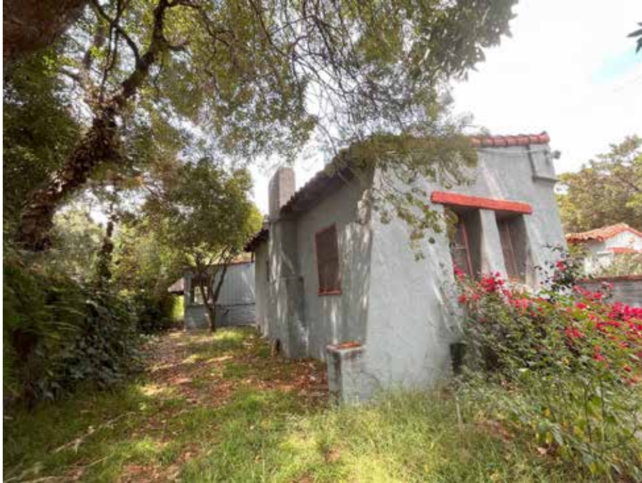
Figure 7. Detail of south and west facing façades, view toward northeast.
