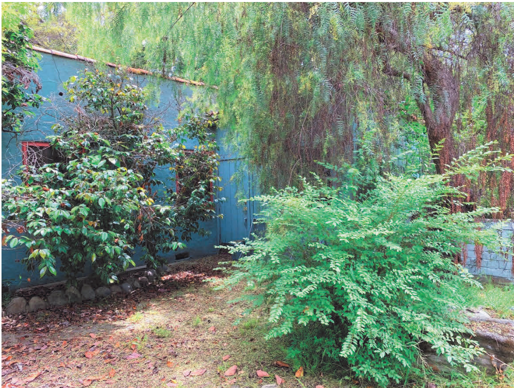
Figure 11. Detail of west façade, view toward northeast.
