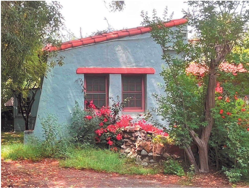
Figure 8. Detail of primary façade windows, view toward north.
