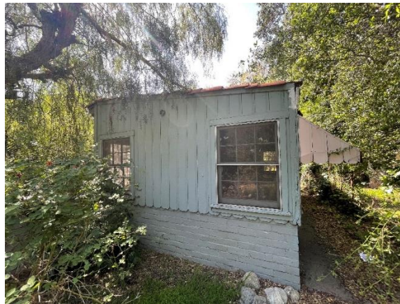
Western Façade (view south)
