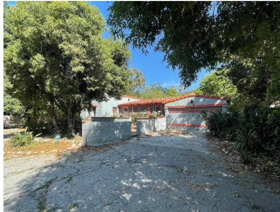
Primary Façade (view northwest)
