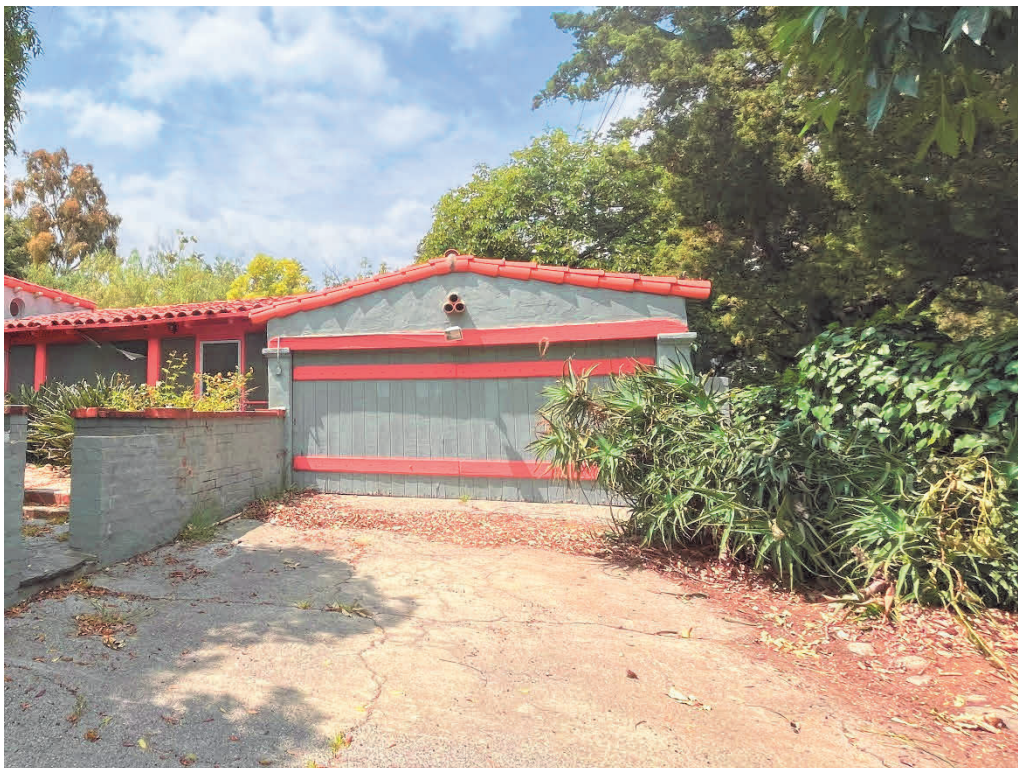
Figure 7. Detail of attached garage, view toward north.
