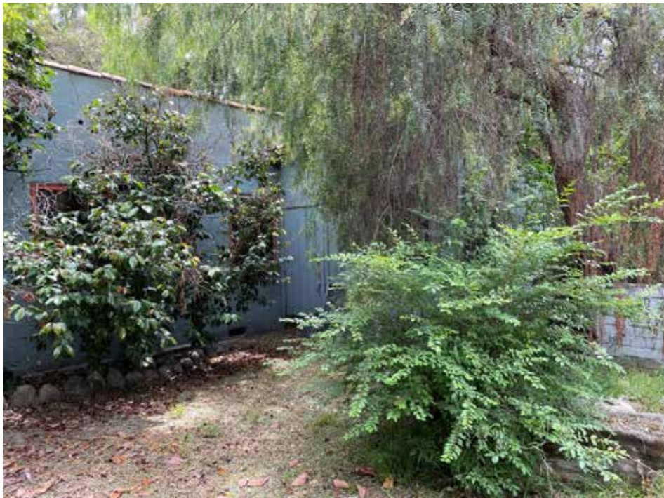
Figure 8. Detail of west façade, view toward northeast.
