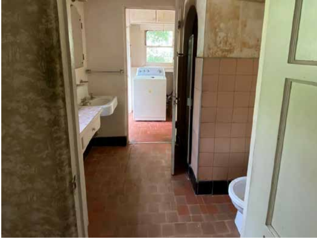
Figure 21. Rear bathroom, view toward east.
