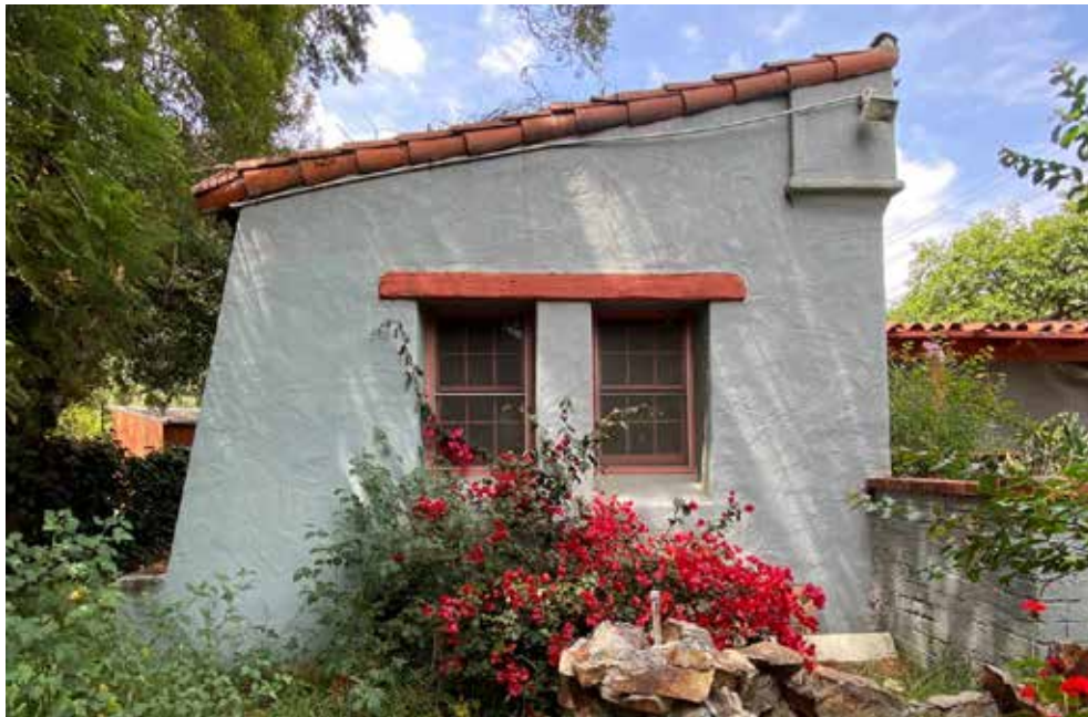
Figure 2. Detail of shed roof section, view toward north.
