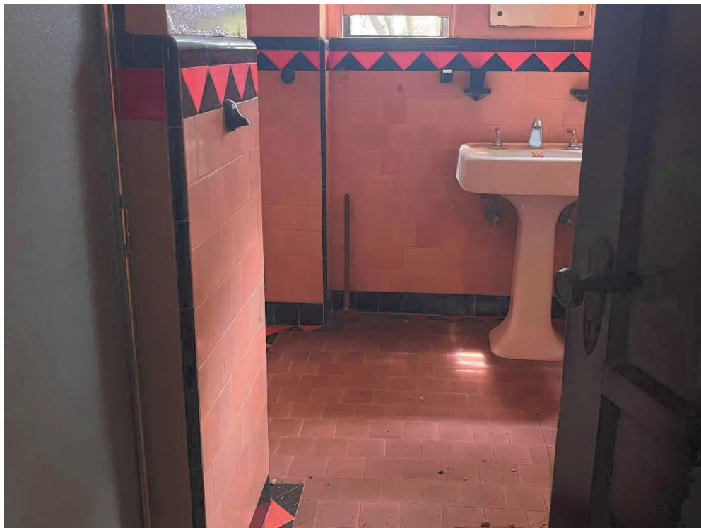
Figure 19. Detail of original tile in bathroom. View toward west.
