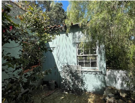
Northern Façade (rumpus room; view west)
