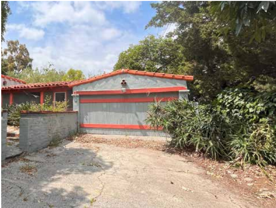
Figure 4. Detail of attached garage, view toward north.
