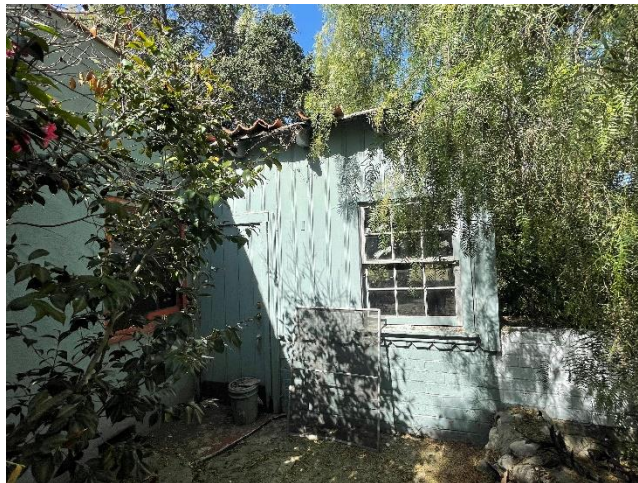
Figure 7E. Northern Façade (rumpus room; view west) SOURCE: Sapphos Environmental, Inc., 2022
