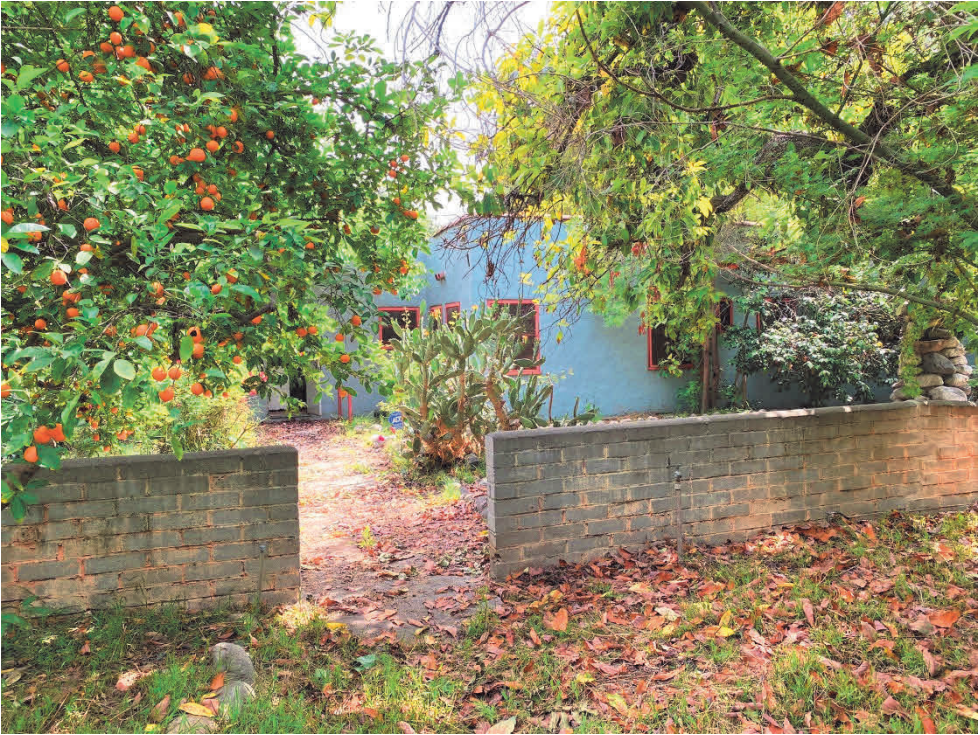
Figure 13. Detail of backyard and concrete wall, view toward south.
