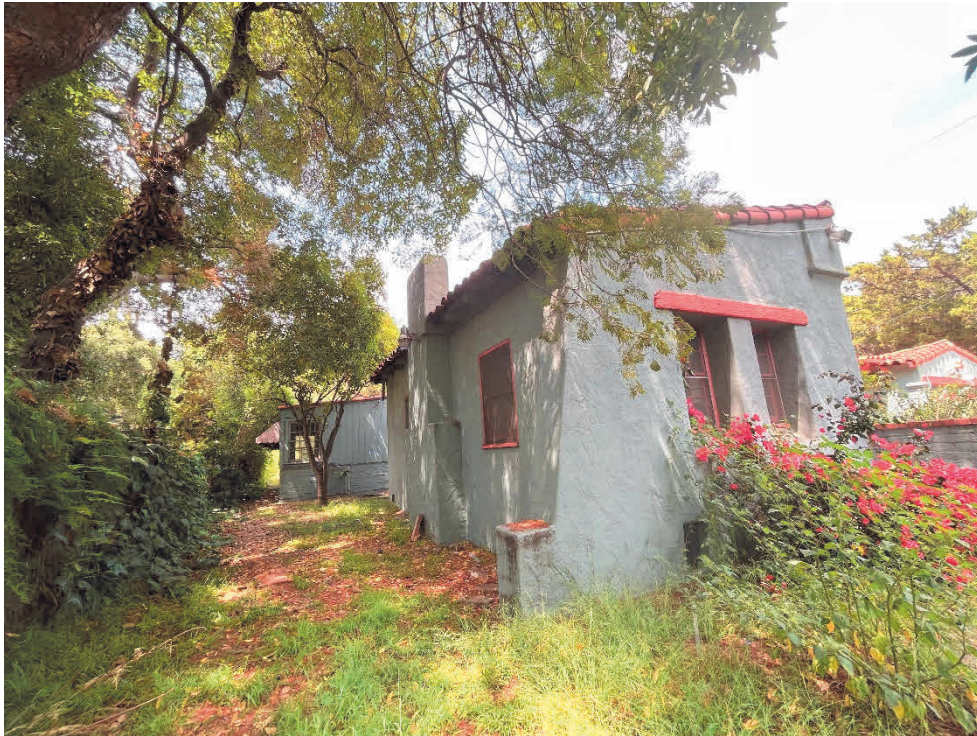
Figure 10. Detail of south and west facing façades, view toward northeast.
