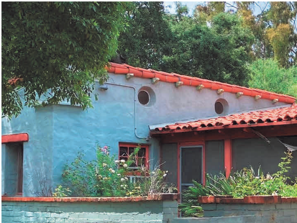
Figure 9. Detail of circular windows along primary façade, view toward northwest
