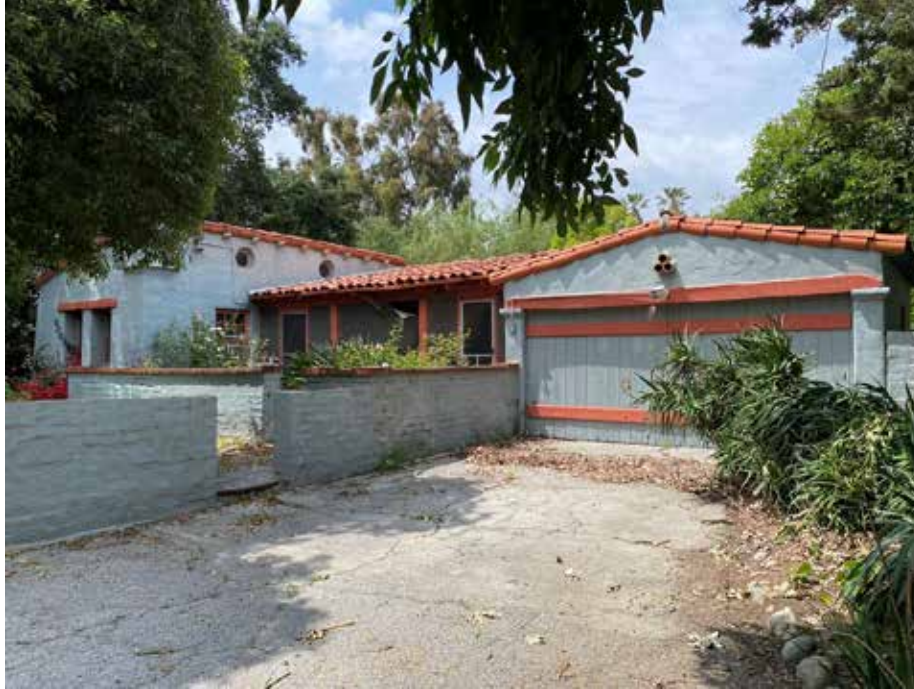
Figure 3. Detail of primary façade, view toward northwest.
