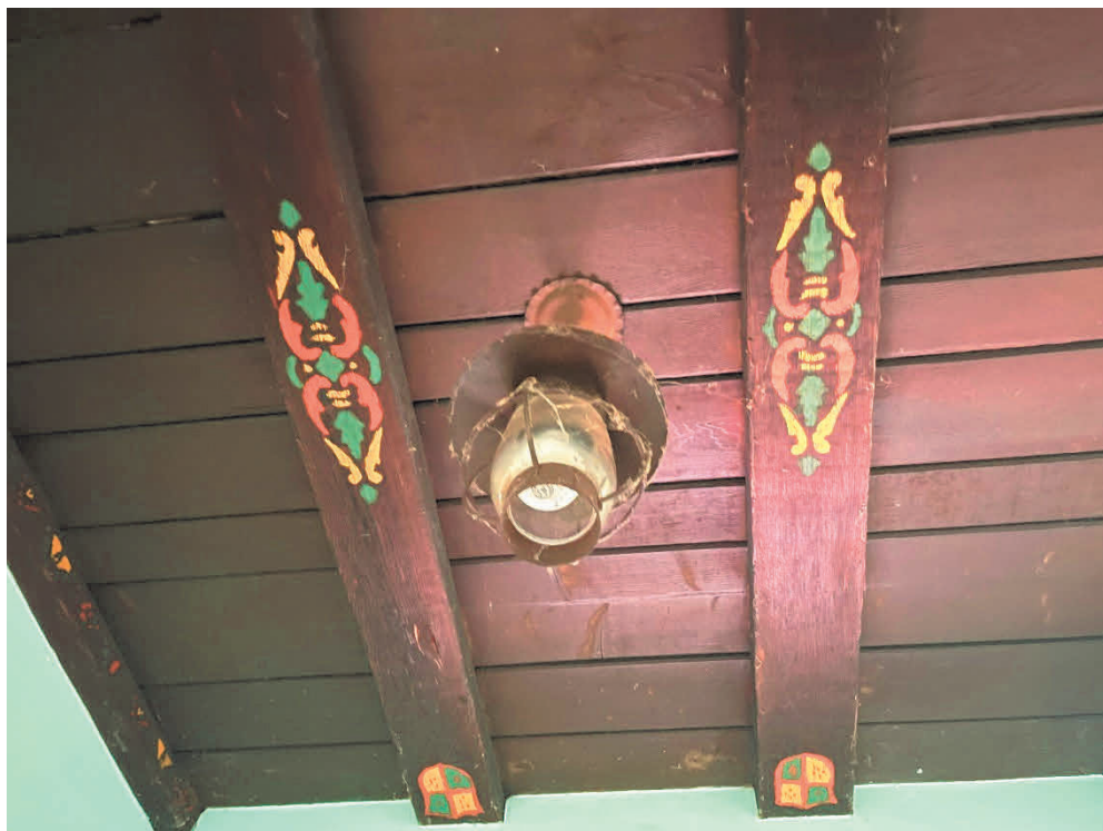
Figure 17. Detail of painted patterns and crests on entrance hall ceiling.
