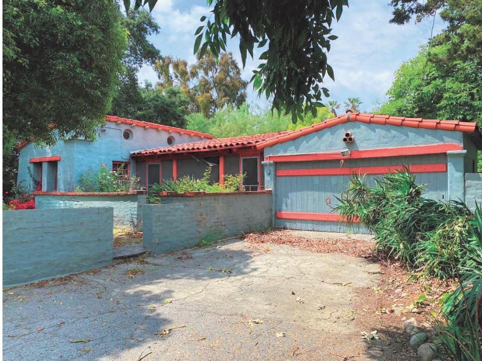
Figure 6. Detail of primary façade, view toward northwest.
