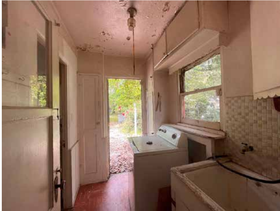
Figure 19. Laundry room and rear exit, view toward north.
