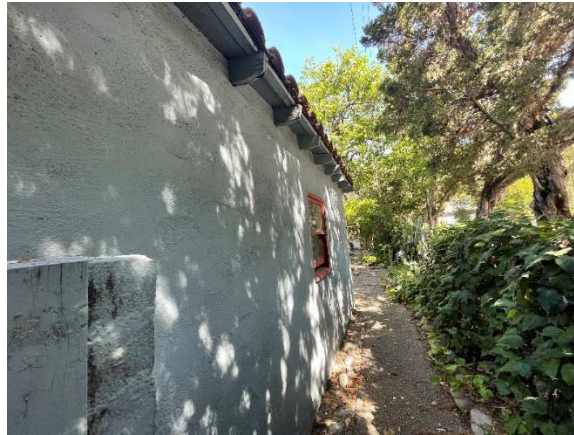
Eastern Façade (view north)
