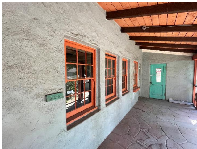
Figure 6C. Primary Façade (porch entryway; view east) SOURCE: Sapphos Environmental, Inc., 2022
