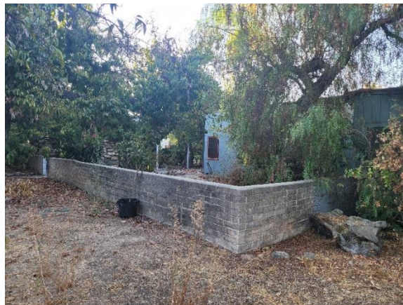
Northern Façade (block wall; view southeast)
