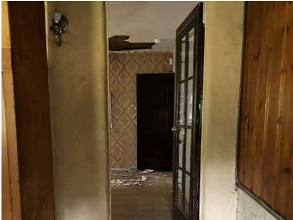
Figure 22. Detail of wooden door into rear bedroom area. View toward south.
