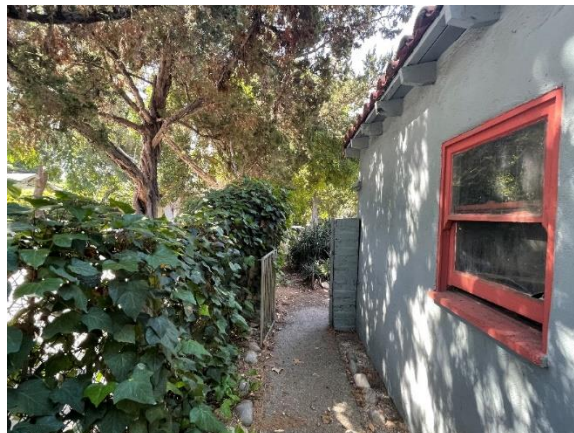
Eastern Façade (view south)
