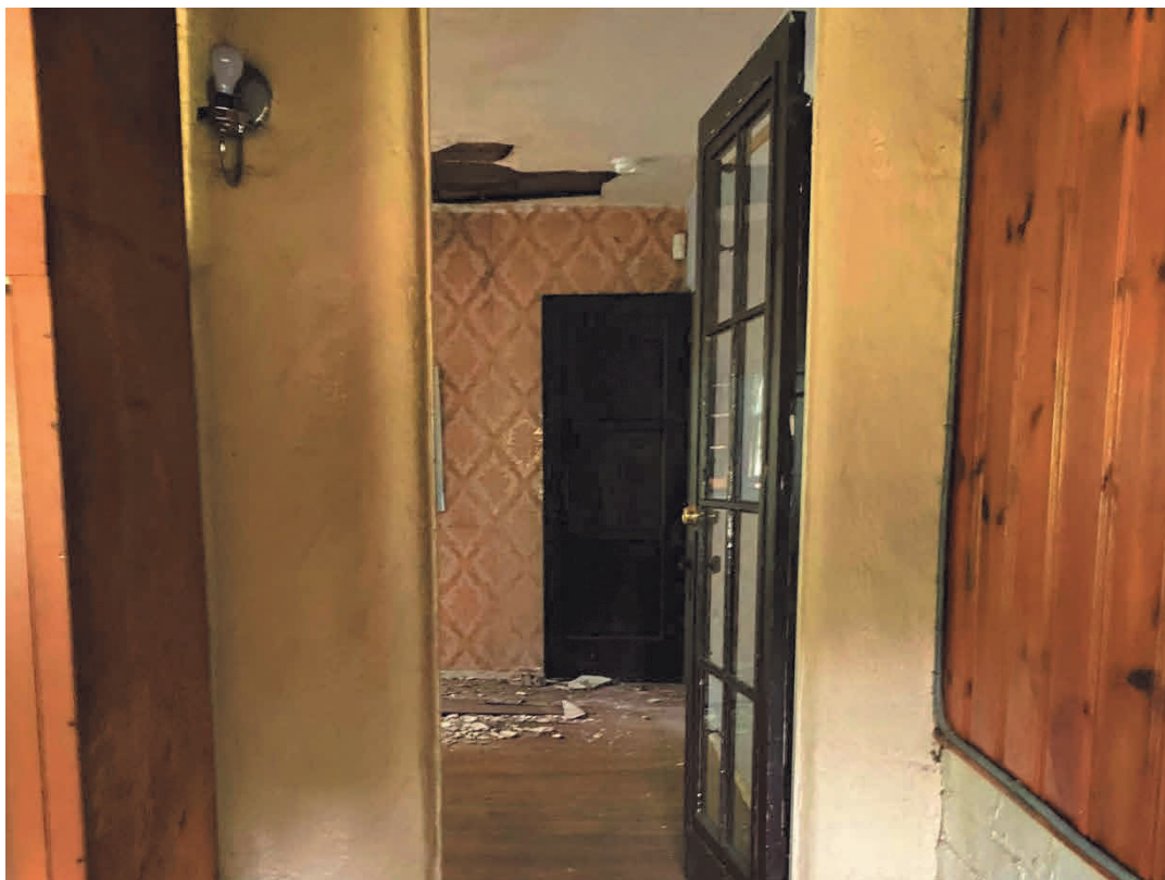
Figure 25. Detail of wooden door into rear bedroom area. View toward south.
