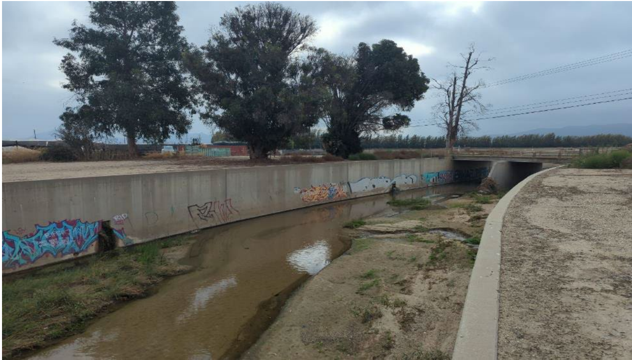
Photograph 1. View of the Revolon Slough in the eastern portion of the Study Area. Note open water in the drainage, as well as patches of sediment accumulation adjacent to open water (Aspect: southeast; September 13, 2023).
