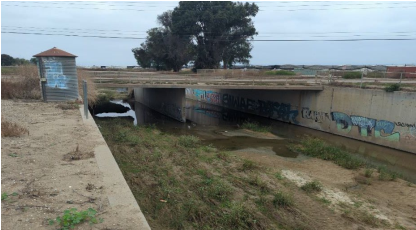
Photograph 3. View of Laguna Road bridge crossing over Revolon Slough, facing northeast.
