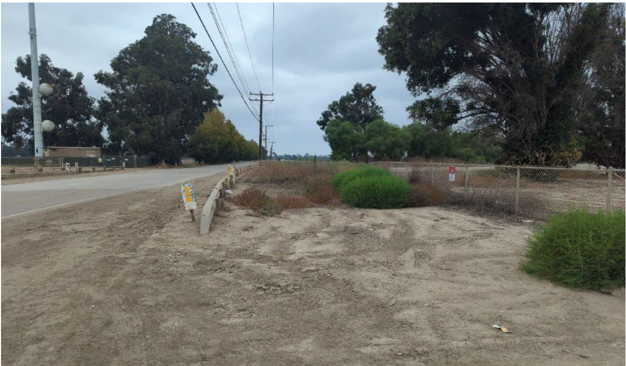
Photograph 10. View of the potential work area above the right (east) bank of Revolon Slough under the North Alignment Alternative (Aspect: west; September 13, 2023).
