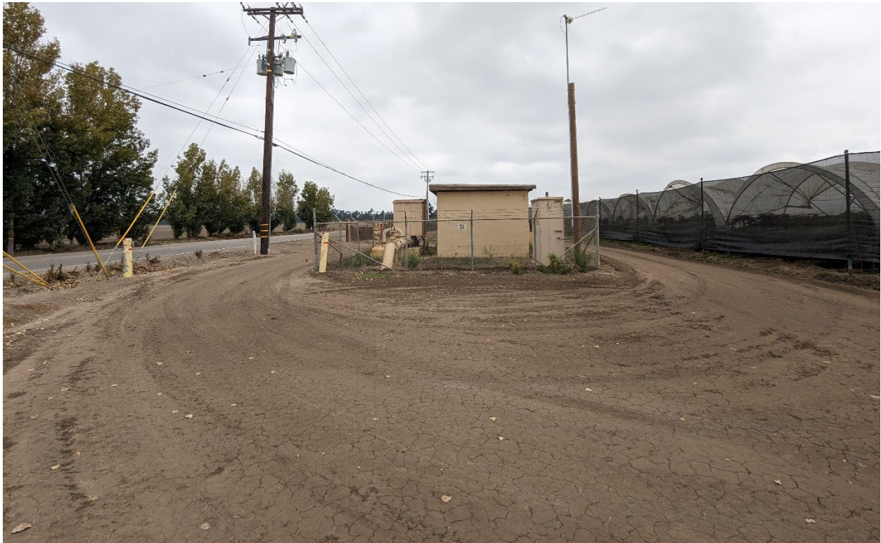
Figure 6 Overview of Project Site Looking West
