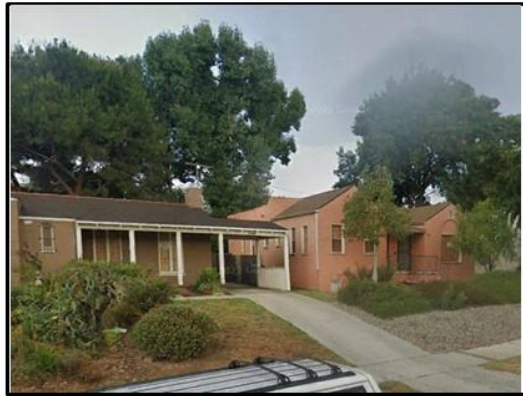
PHOTO 1: View of the northern portion of the project site along Sheffield Avenue.
