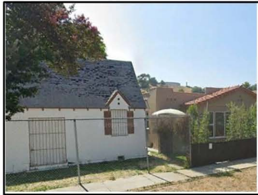
PHOTO 1: View of the northern portion of the project site along Maycrest Avenue.
