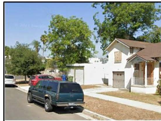
PHOTO 2: View of the north-eastern portion of the project site along Almont Street.
