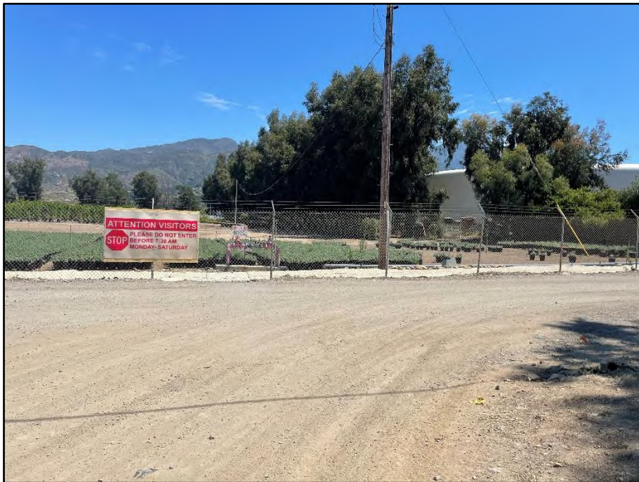
Figure 6. Overview of Location 4, view facing north.
