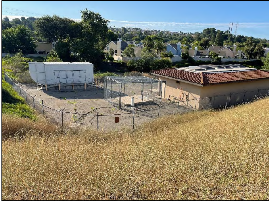
Figure 3. Overview of Location 1, view facing east
