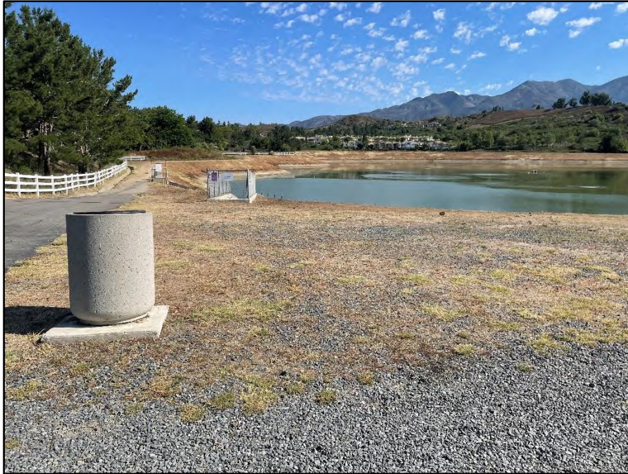
Figure 5. Overview of Location 3, view facing north.
