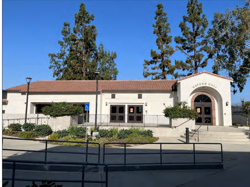
Hayden Hall (HH), east elevation, facing west.
