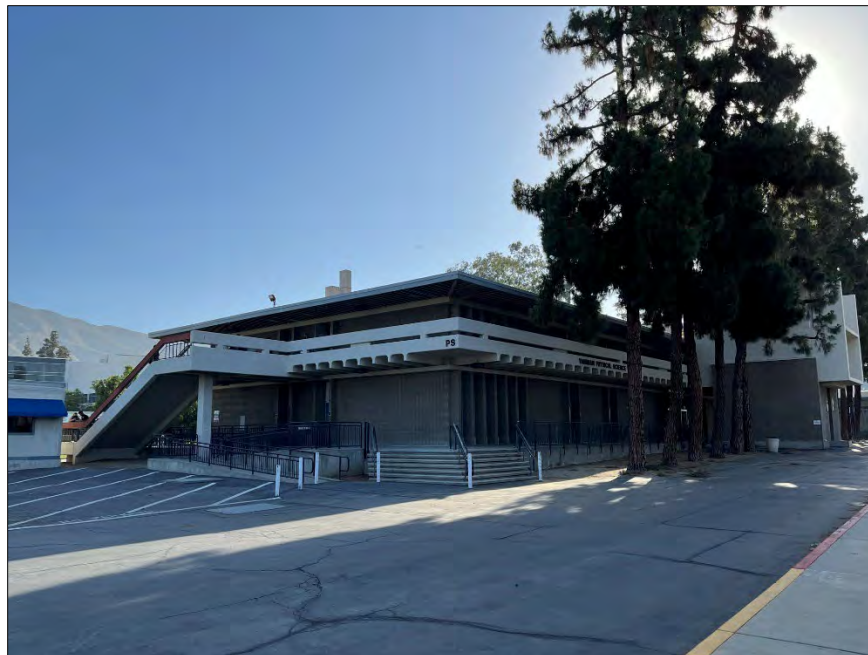
Physical Science (PS), south and west elevations, facing southeast.
