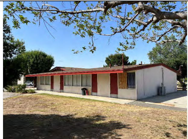
East and north elevations, facing southwest
