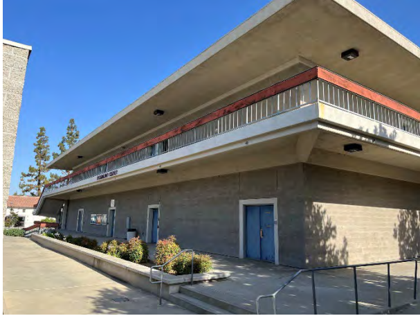
South elevation, facing northwest
