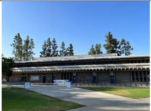
North elevation, facing southeast
