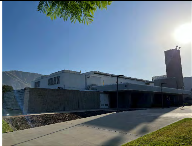
South and west elevations, facing northeast
