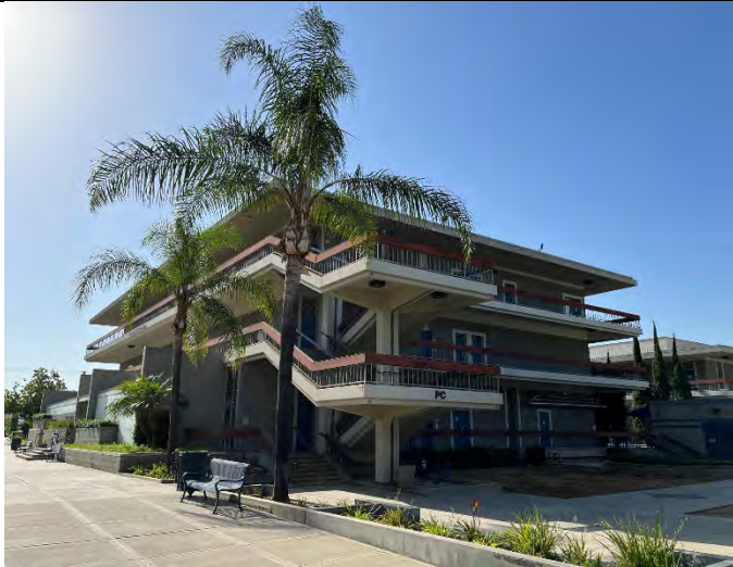
North and west elevations, facing southeast
