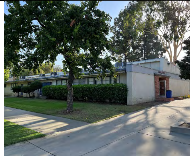
South and west elevations, facing northeast
