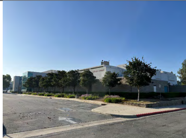
North and west elevations, facing southeast
