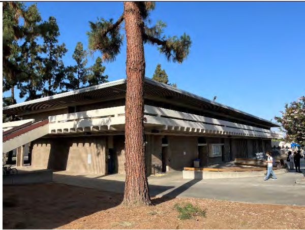
North and east elevations, facing southwest
