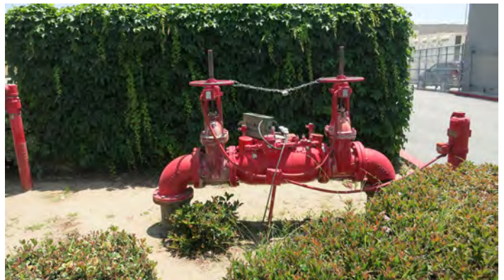
Noise Measurement Site 3 - looking south
