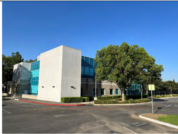
East addition, facing southwest
