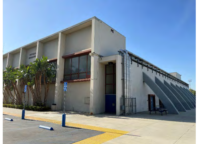
North and west elevations, facing southeast
