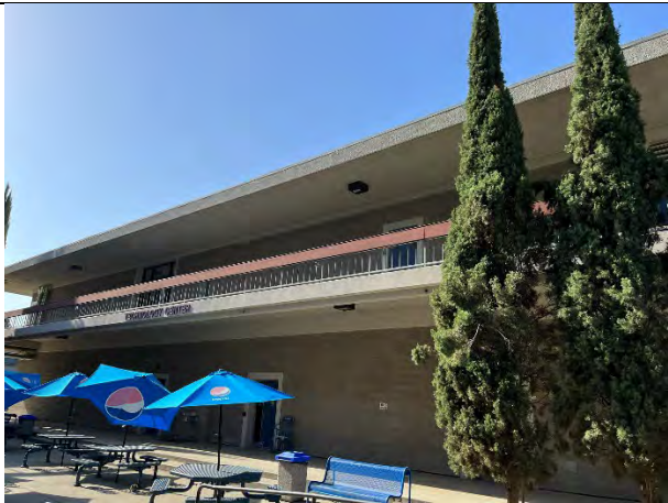
North elevation, facing southeast
