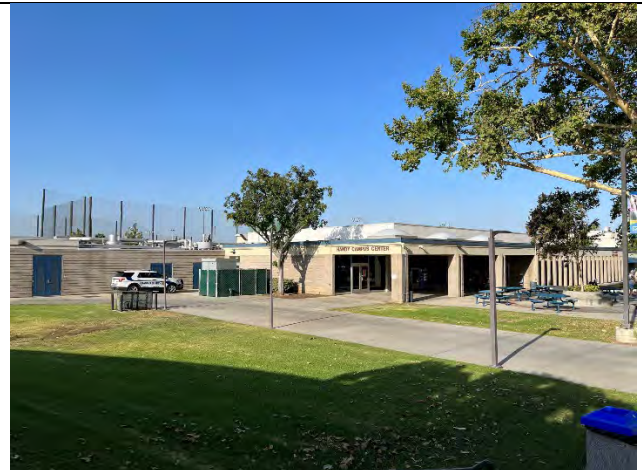
East elevation, facing southwest
