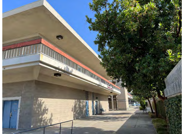
East elevation, facing northwest
