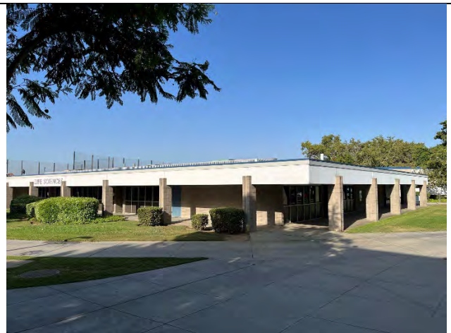
North and east elevations, facing southwest
