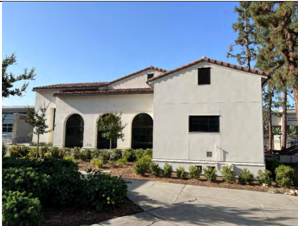
North elevation, facing south
