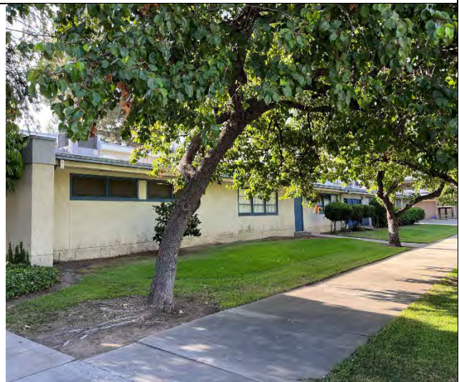
West elevations, facing southeast
