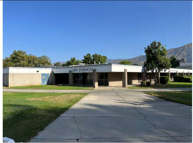
South and east elevations, facing northwest
