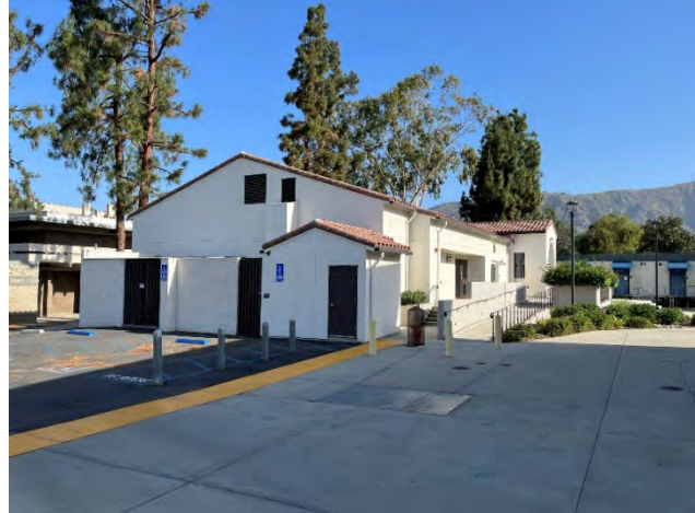
South and east elevations, facing northwest
