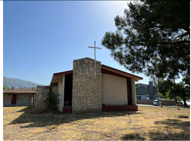
west elevation, facing east
