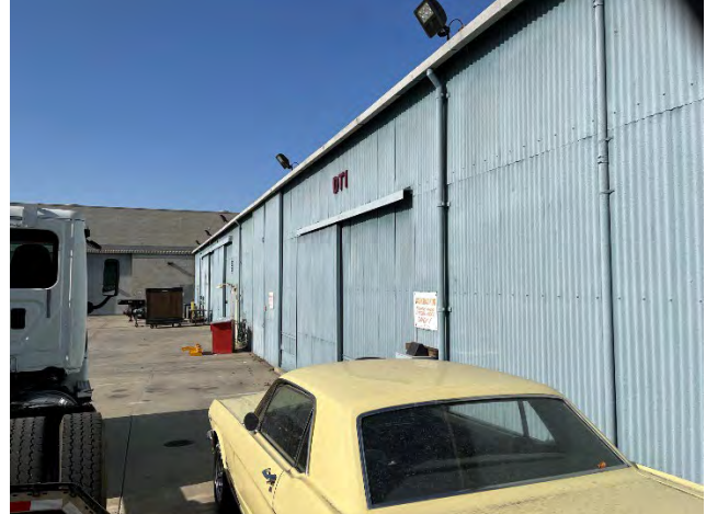
East elevation, facing southwest
