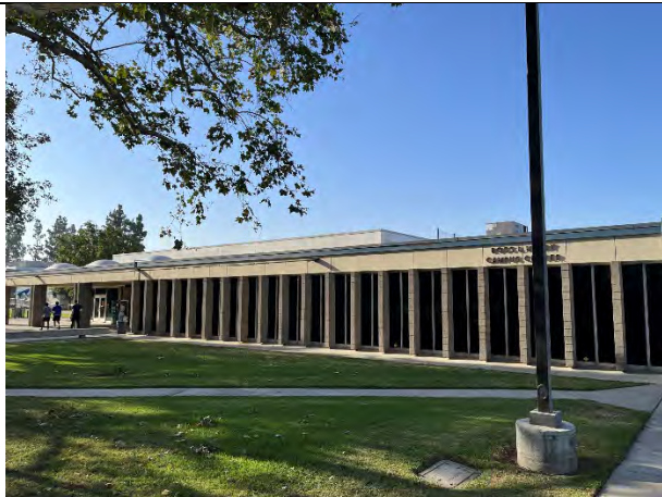
North elevation, facing southeast
