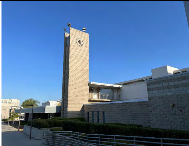
South elevation, facing northwest
