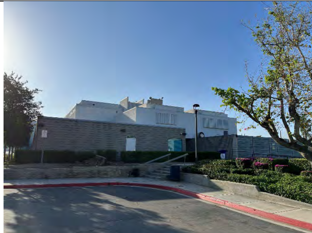
West elevation, facing east
