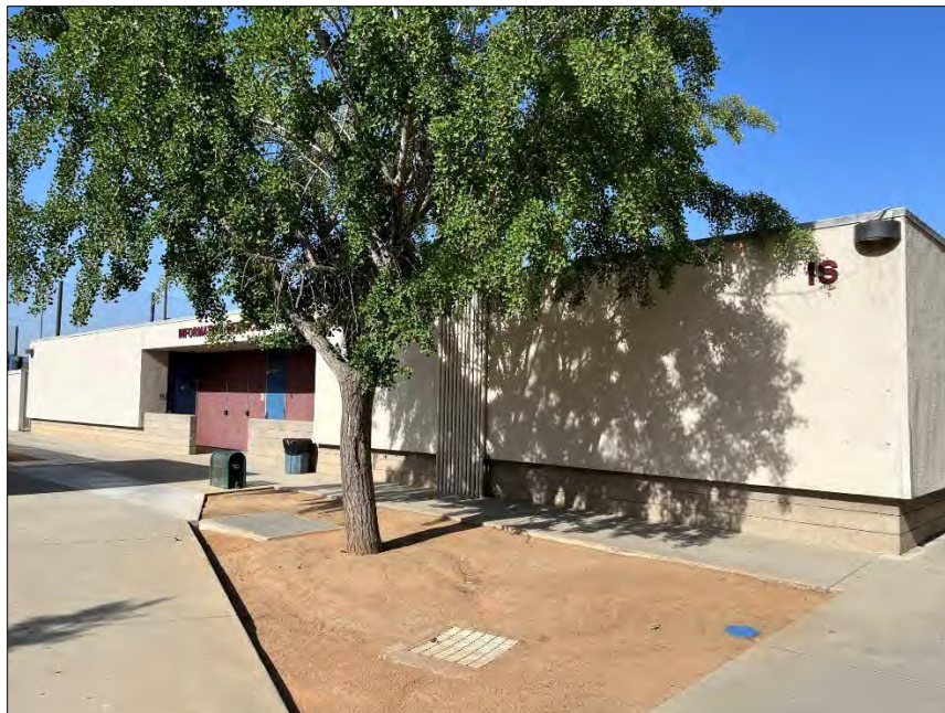
Information Services (IS), east elevation, facing southwest.
