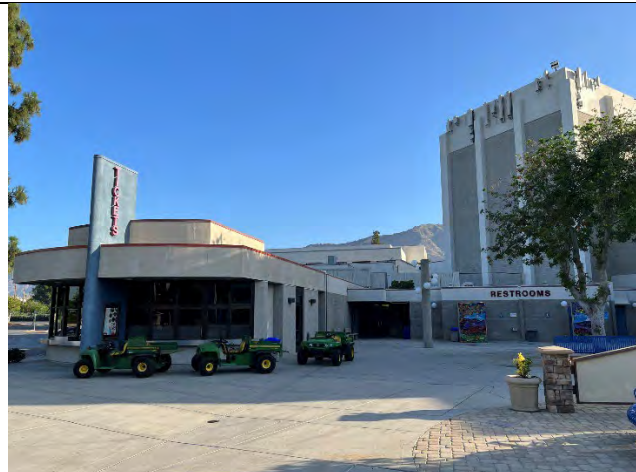
South and west elevations, facing north
