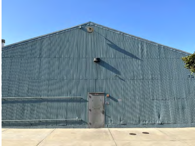
North elevation, facing south
