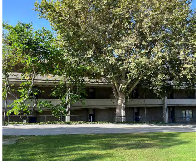
North elevation, facing south
