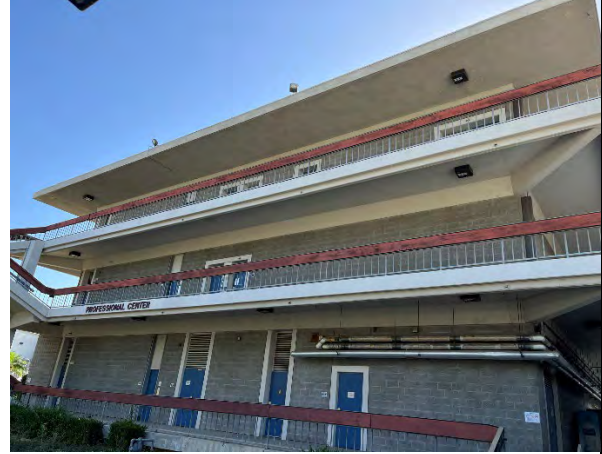
West elevation facing east
