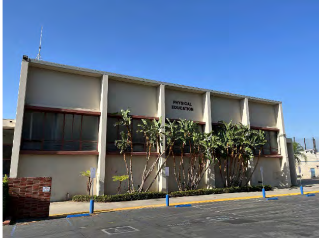
North elevation, facing south
