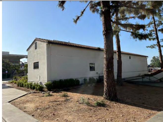
North and west elevations, facing southeast
