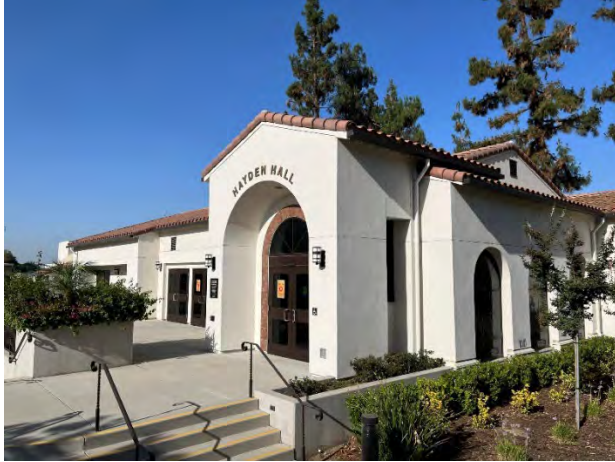
North and East Elevations, facing southwest
