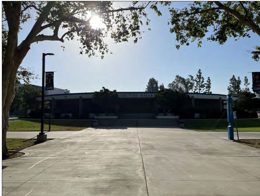
Lecture Hall/Life Science (LH/LS), west elevation, facing east.
