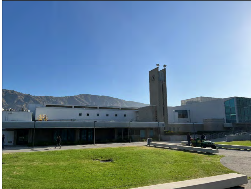
Hayden Library (LI), south elevation, facing northeast.
