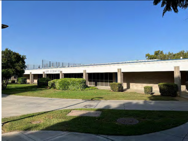
east elevation, facing southwest
