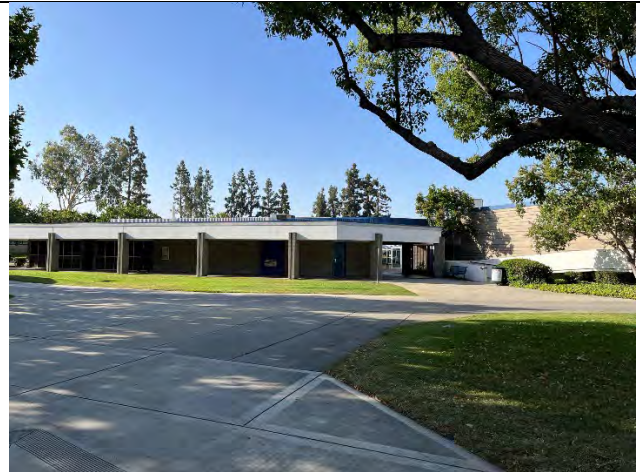
North elevation, facing south
