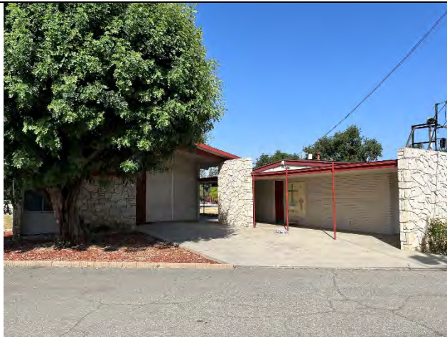
East and south elevations, facing northwest
