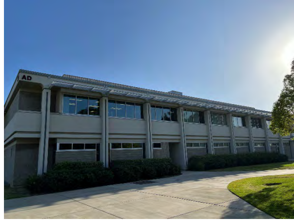
South elevation, facing southeast
