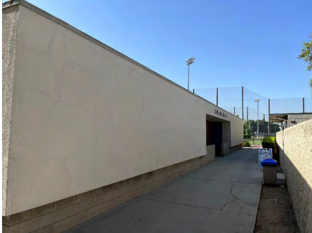
West elevation, facing southeast
