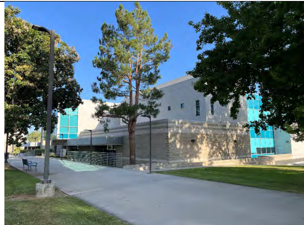
East addition, facing northwest
