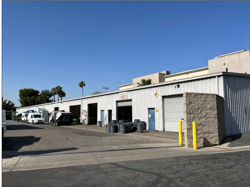
Maintenance & Operations Warehouse (MO/WA), east elevation, facing southwest.
