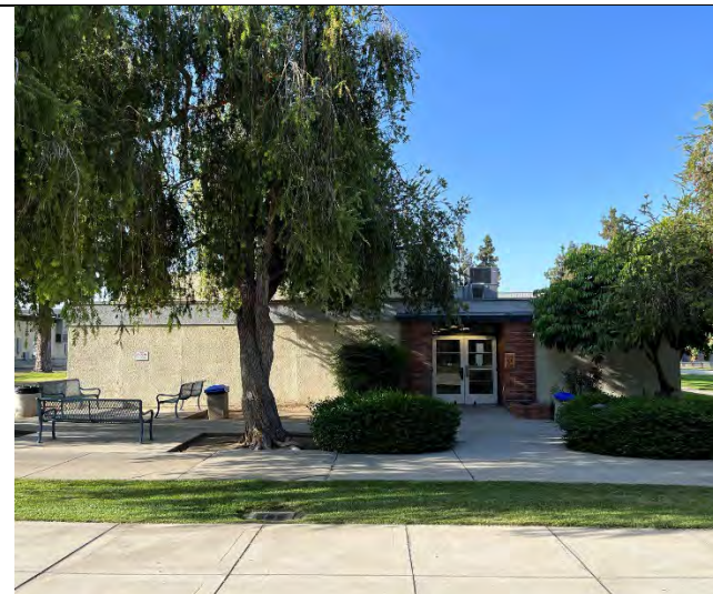
North elevation, facing south
