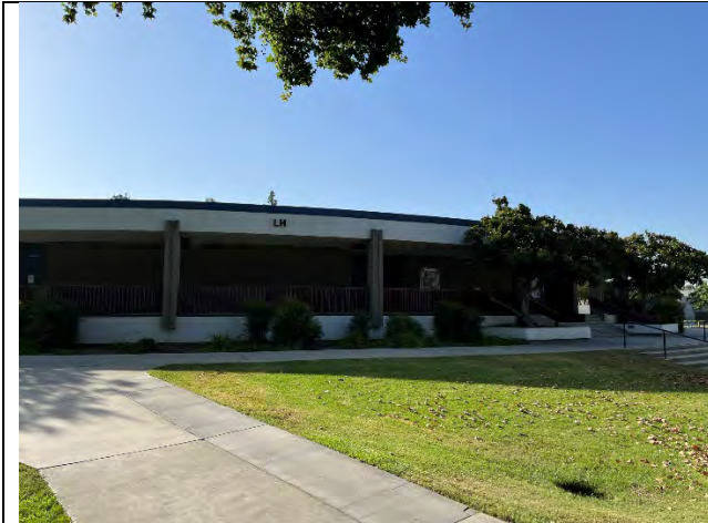
West elevation, facing southeast
