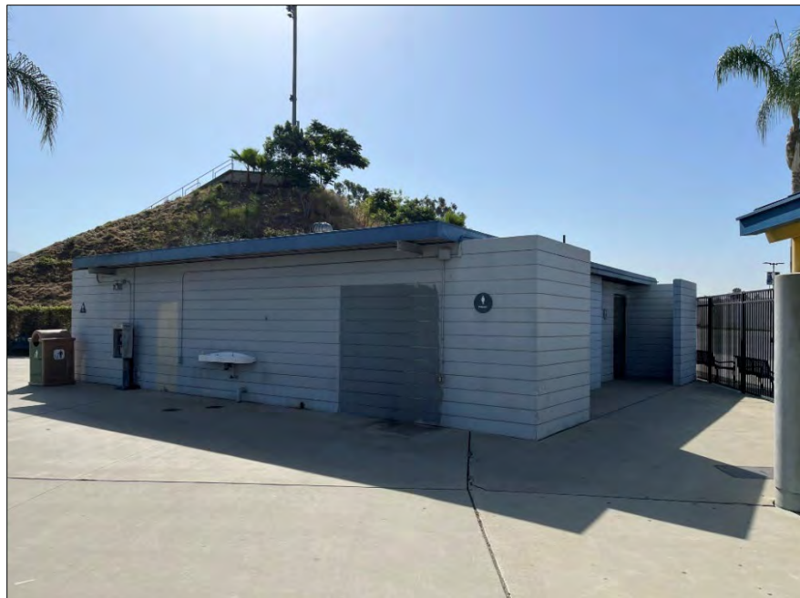
South Stadium Restroom (SSRR), south and west elevations, facing northeast.
