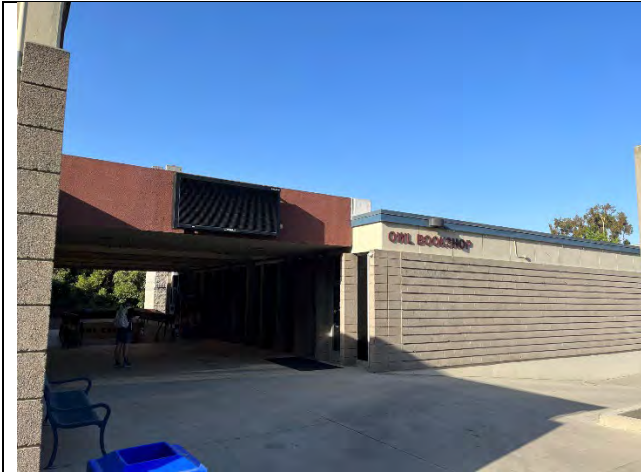
North elevation and courtyard, facing southwest
