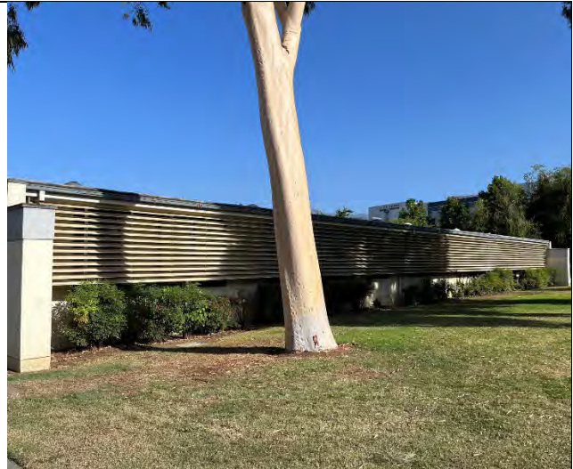
East elevation, facing northwest
