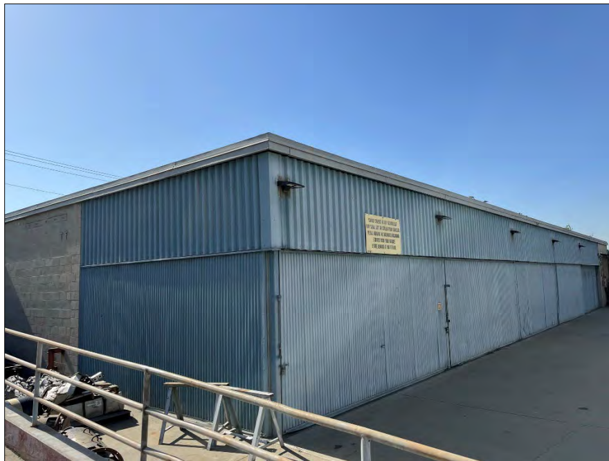
Automotive Annex (AA), west elevation, facing southeast.
