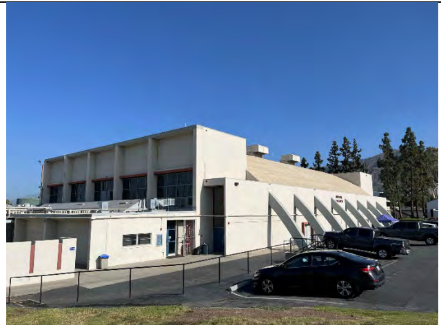
South and east elevations, facing northwest
