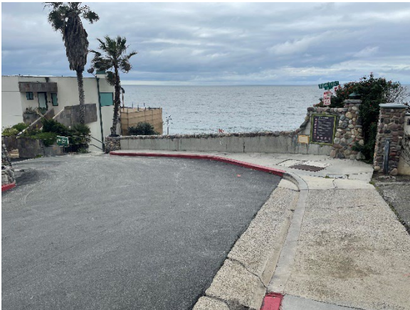
Photograph 3: View of concrete wall at top of Cleo Street beach access stairs, looking west (Stantec, March 2023)
