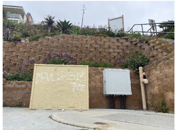
Photograph 4: View of concrete block retaining wall and concrete pad (Stantec, March 2023)
