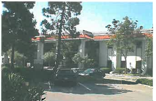
Photo #28: Commercial/office facility adjacent to south of Project
