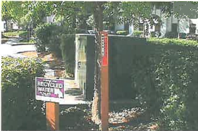
Photo #27: Gas pipeline warning post and electrical equipment box on southeast corner of Project site
