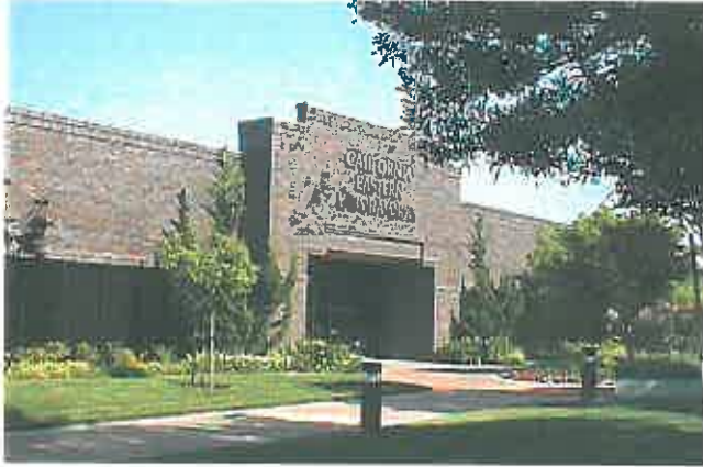
Photo #1: Front (east) elevation of Project building
