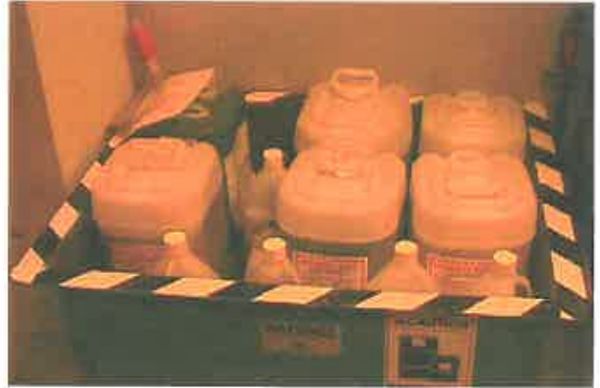
Photo #14: Hazardous waste storage area in double containment in PCB Etch Room
