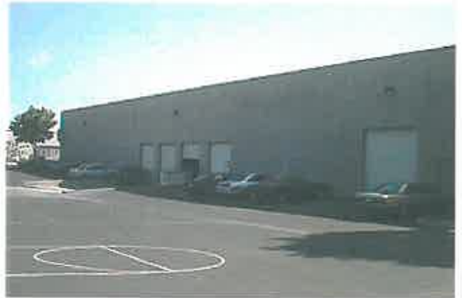
Photo #2: Rear (west) elevation of Project building
