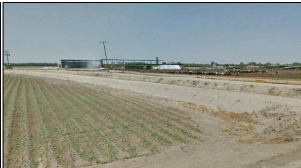
Photo 2: Northeastern Site Boundary (View Southwest)
