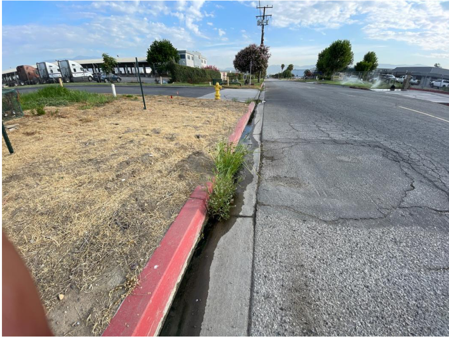
Photo 7. View of concrete street gutter near the eastern boundary of the project site with standing water and hydrophytic vegetation; this area is not anticipated to be a jurisdictional aquatic resource (see Section 3.5).
