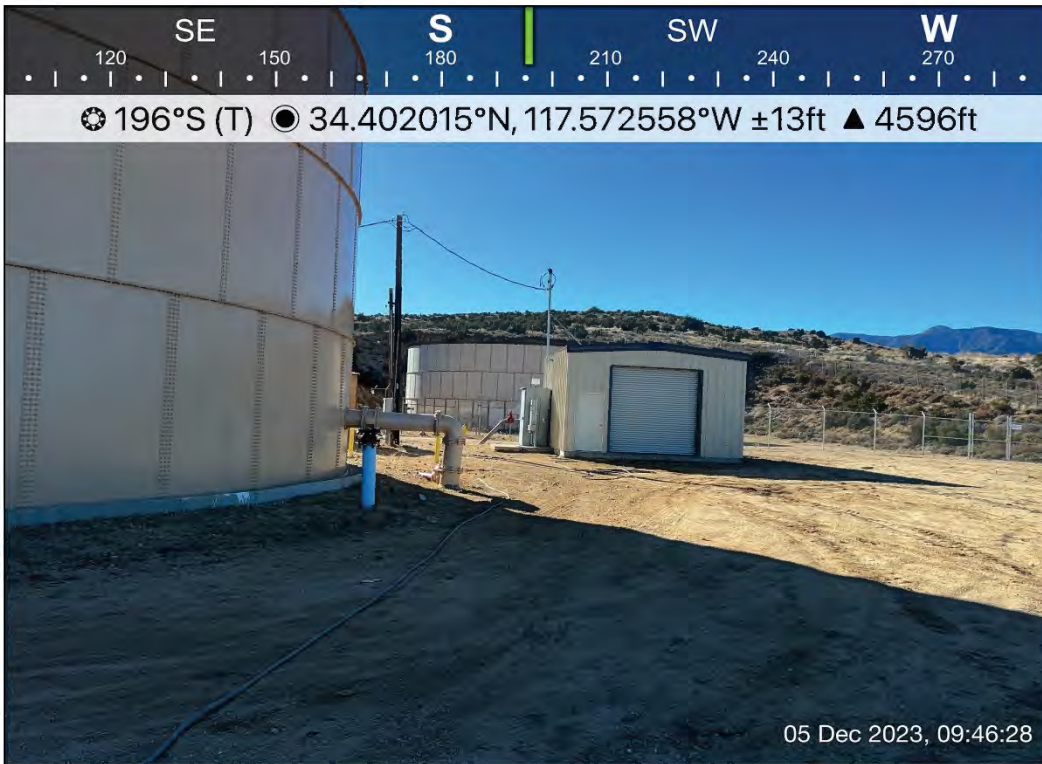
Photo. View of existing Reservoir 6A
