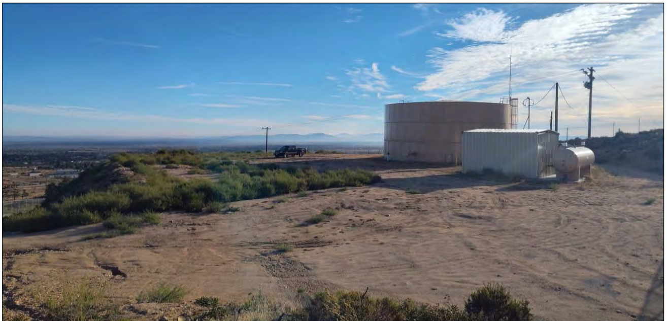
Figure 4. Current natural setting of the APE. (Photograph taken on September 22, 2023; view to the northeast)
