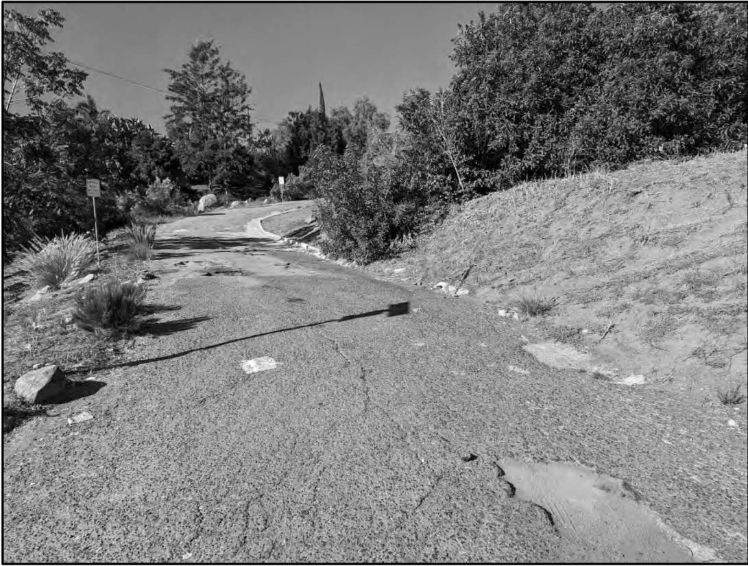
Photo 3. View facing west from the southeast corner of the property showing site access from Cajon View Drive.
