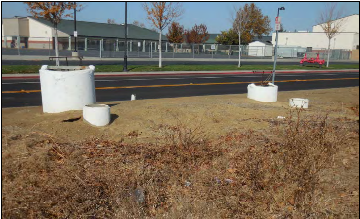
Figure 7: Irrigation valves/concrete risers, northwest corner of the parcel (Adams Lane in background)
