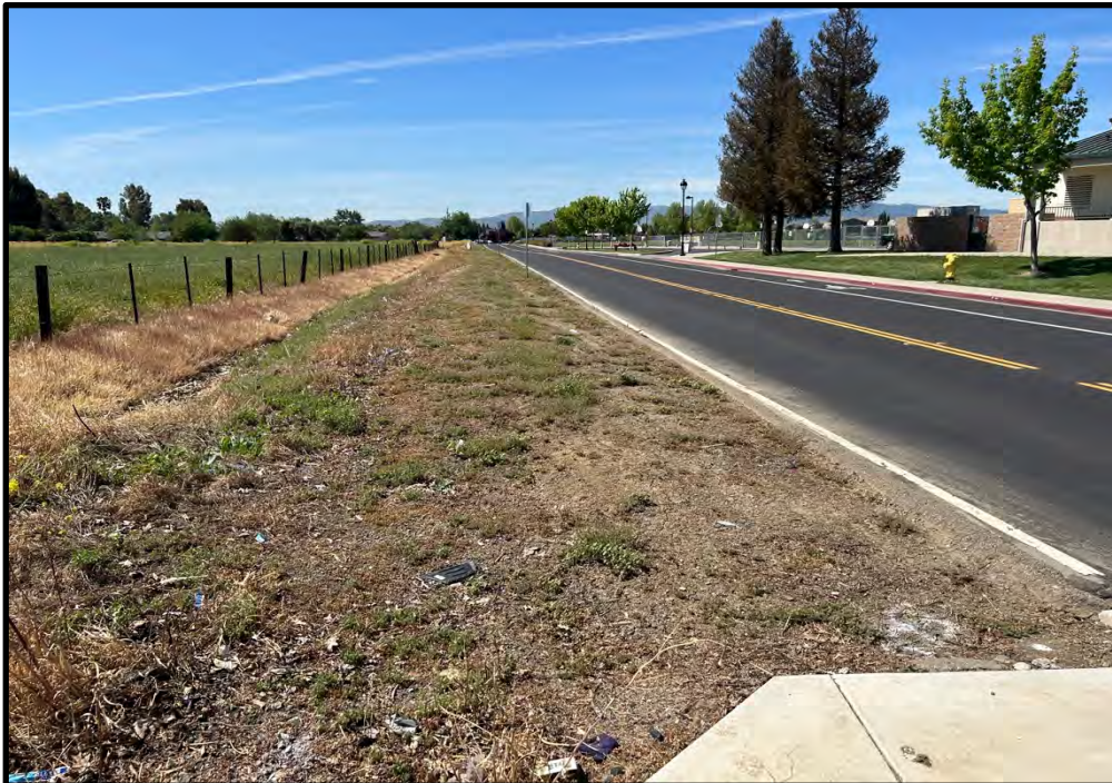
Shoulder of Adams Lane adjacent to the west edge of the site, looking southwest; 04/28/23. This area will be subject to off-site road and/or shoulder improvements as part of the project.
