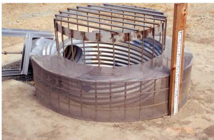
Figure 1 Example of Extended Detention Outlet Structure
