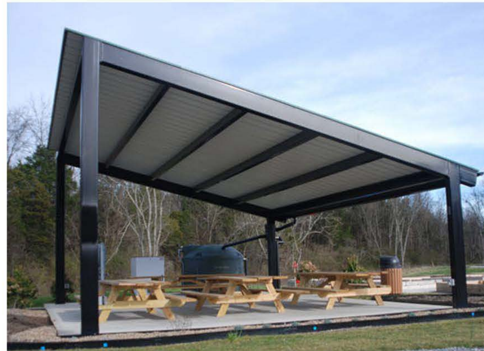
SOLID ROOF MONOSLOPE STEEL STRUCTURE
