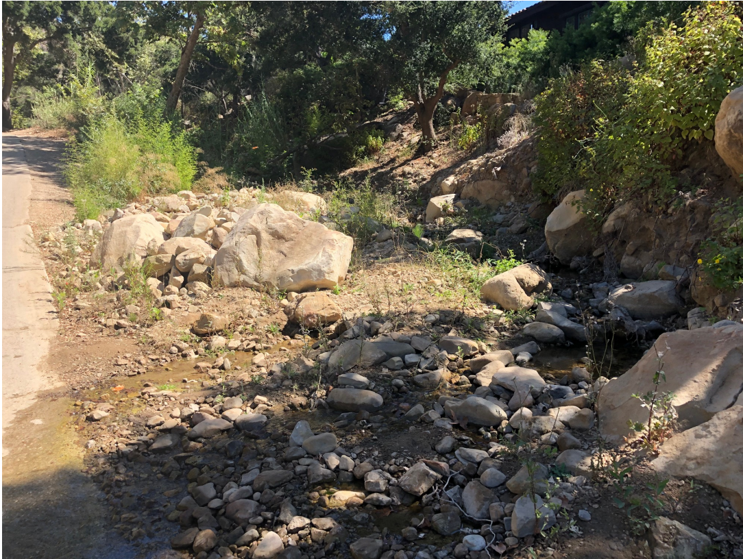
Photo 3. Montecito Creek on East Side of Crossing, Facing Northeast.
