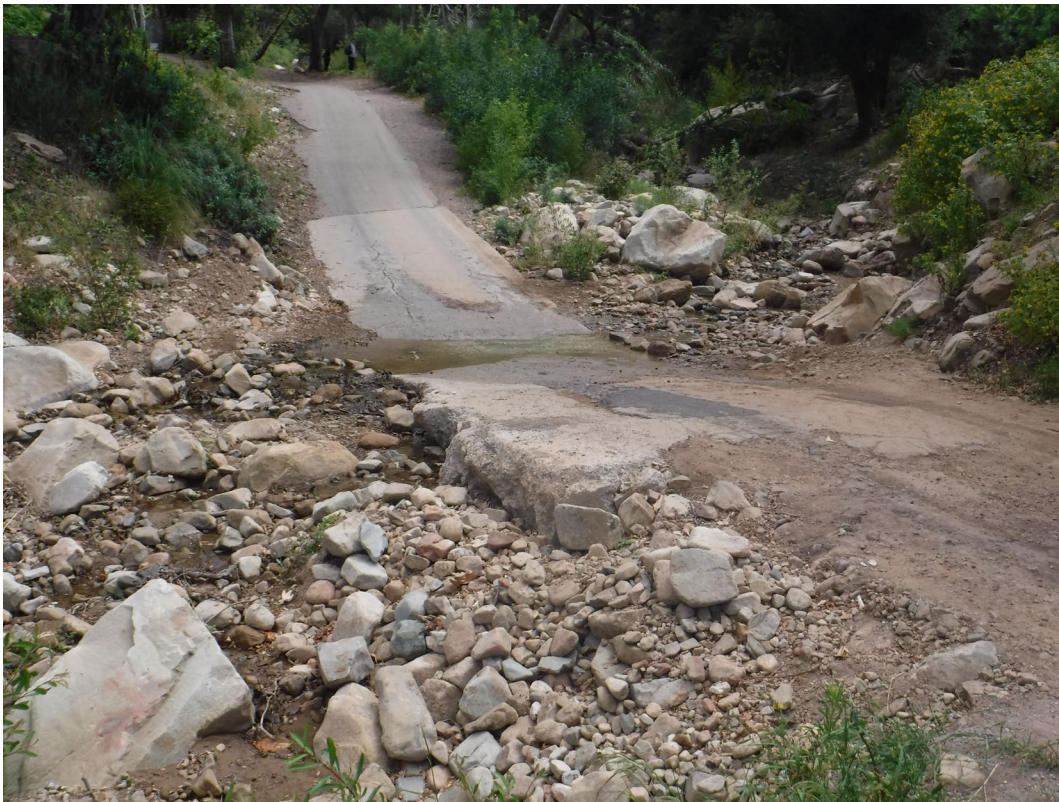
At-grade crossing, looking upstream. Bed gradient steepens significantly immediately downstream of crossing (at left).
