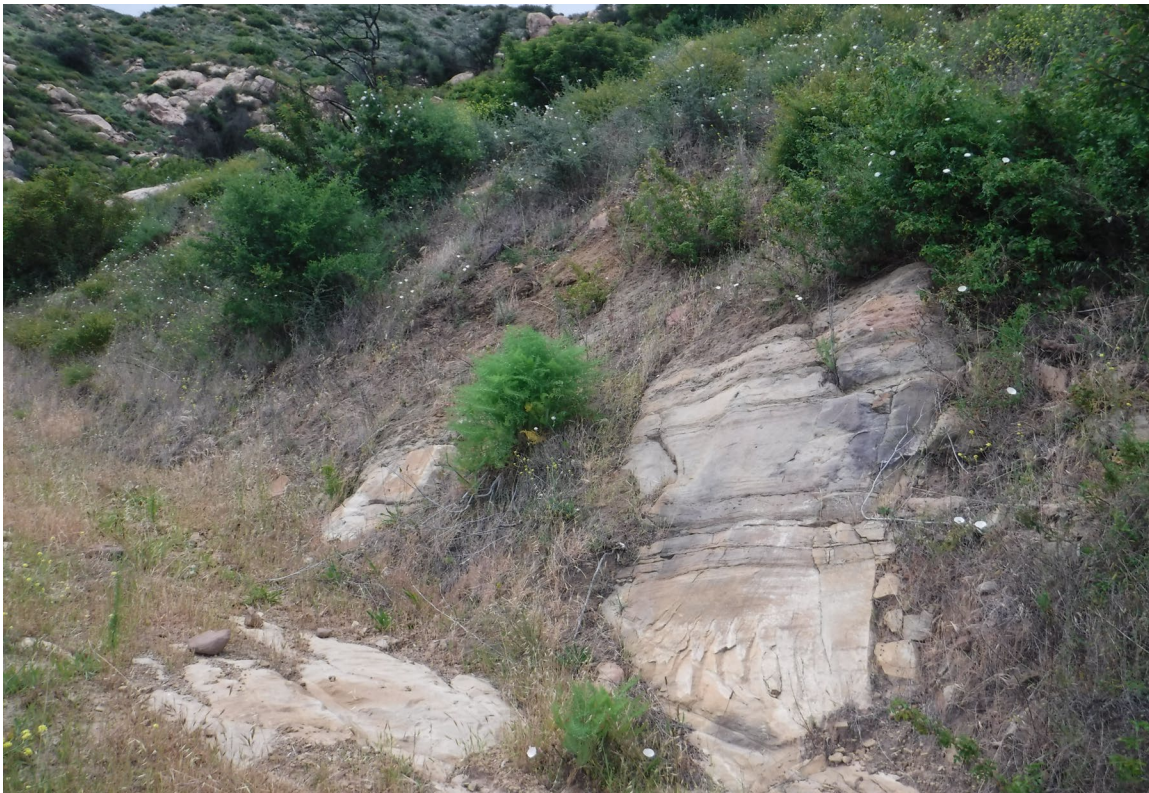
Access road near Station 31+00, showing re-growth of diverse coastal sage scrub vegetation.
