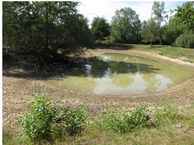
Infiltration pond in a natural area. The infiltration portion consists of sand with a high infiltration rate.
