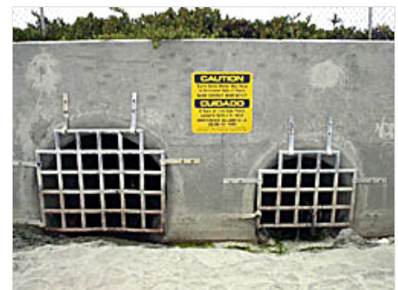
Stormwater Outlet at a Coastal Beach
