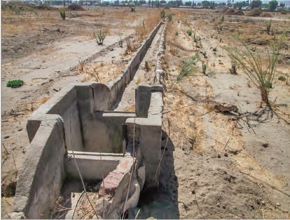
View south of flume showing brick-and-mortar weir (flow control structure)
