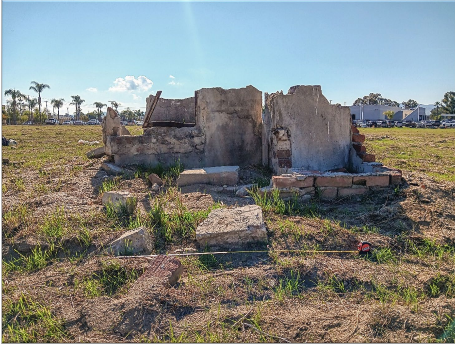
Photograph 7: Feature A, view to the south.
