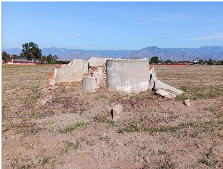
Photograph 8: Feature A, view to the north.
