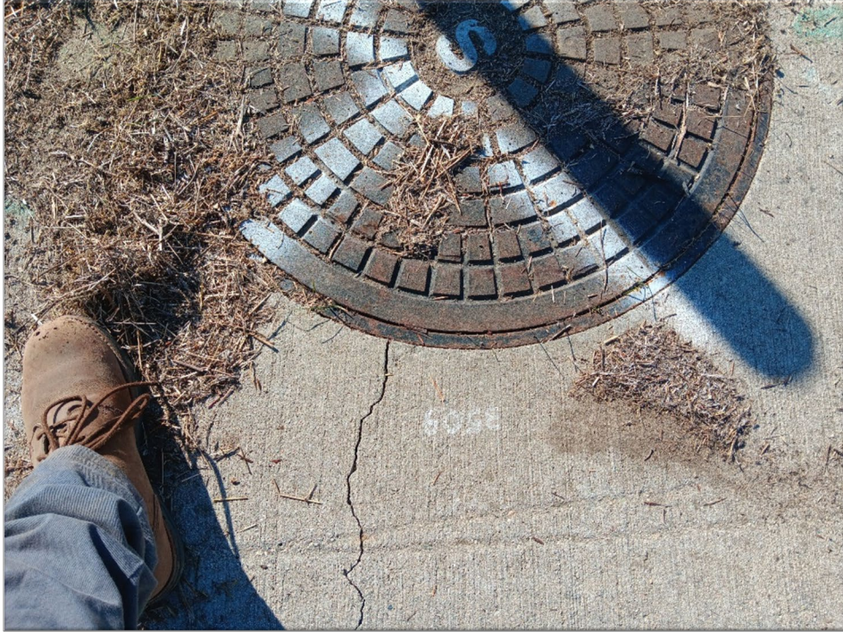
Photograph 5: Underground wastewater underground line, plan view.
