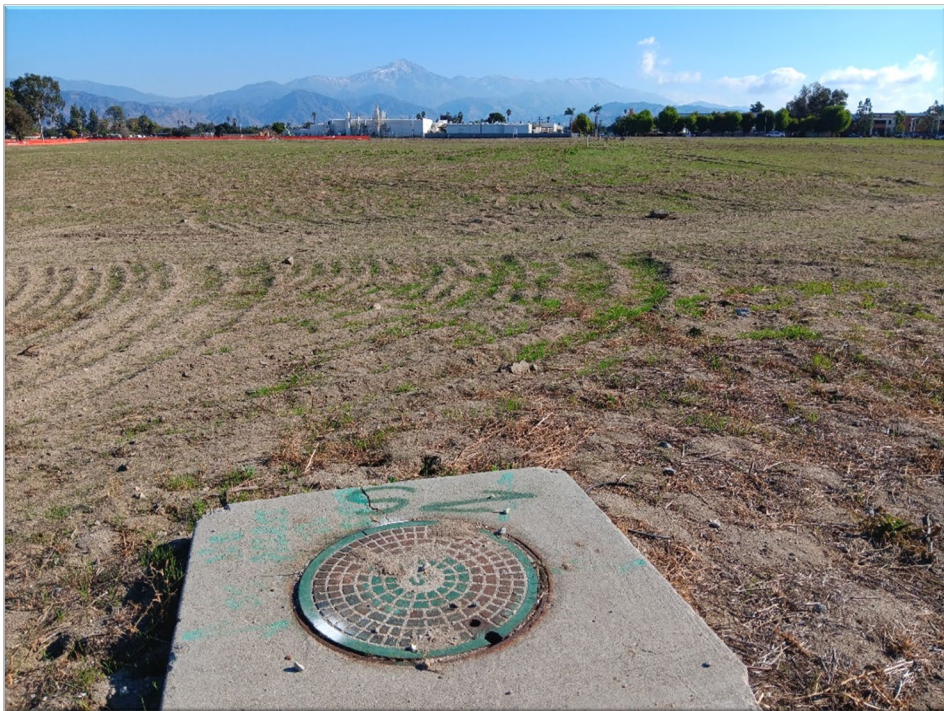
Photograph 6: Underground wastewater line, alignment to the east, view to the east.
