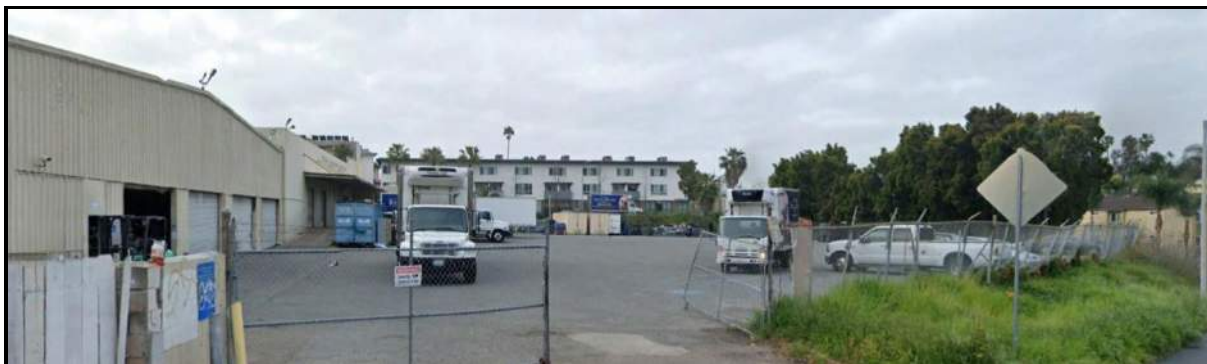
Figure 4-2. Site Surface Conditions, Viewed from the North
