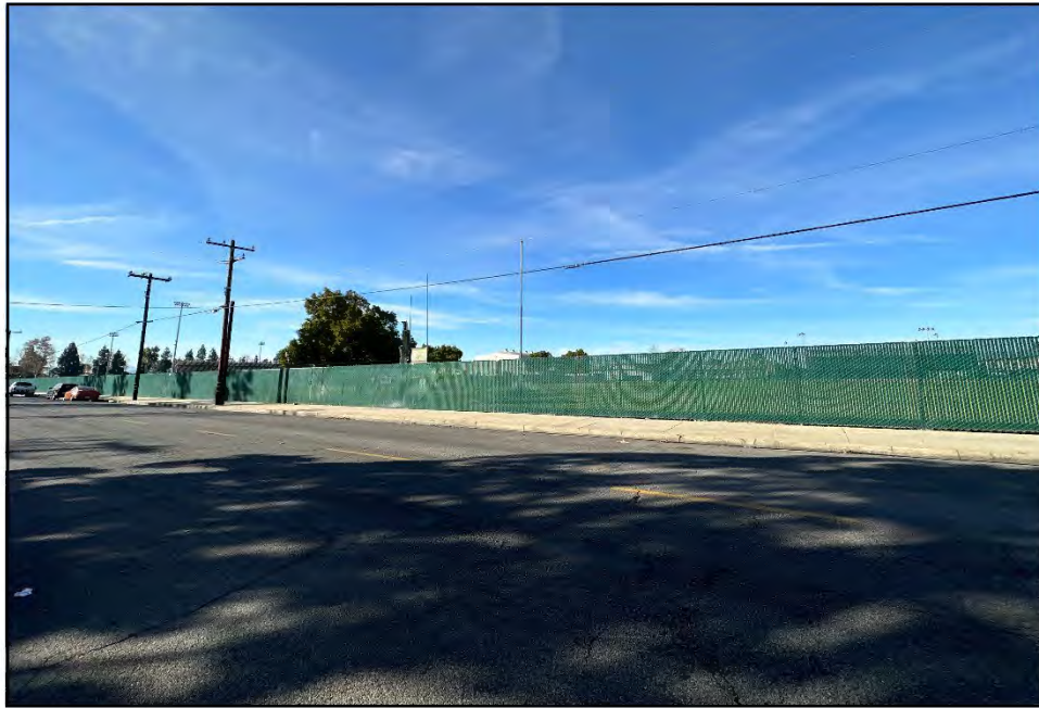
Photo 2. Looking west towards the Project Site from across North Willow Avenue.
