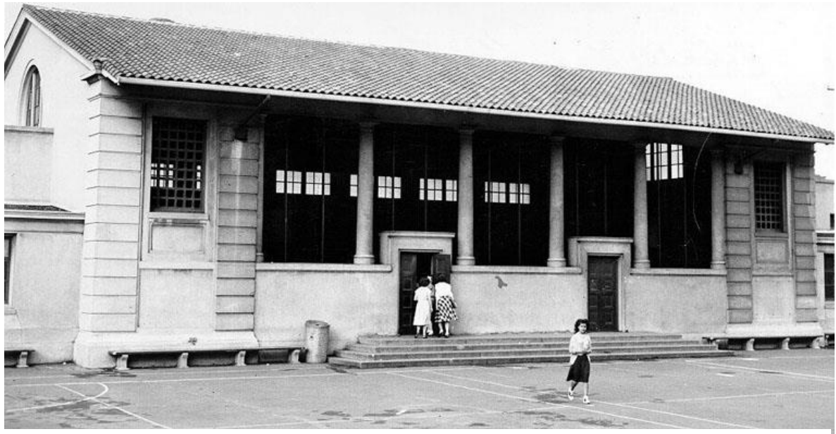
The east façade of the original gym wing had an open colonnade, and the smaller openings flanking it had unglazed wood grilles. San Francisco Public Library.
