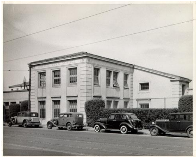
Shop wing from Valencia Street, looking northeast. Several original windows and the shed-roofed extension on the right seen here have been removed, along with the hedge at the street. San Francisco Public Library.
