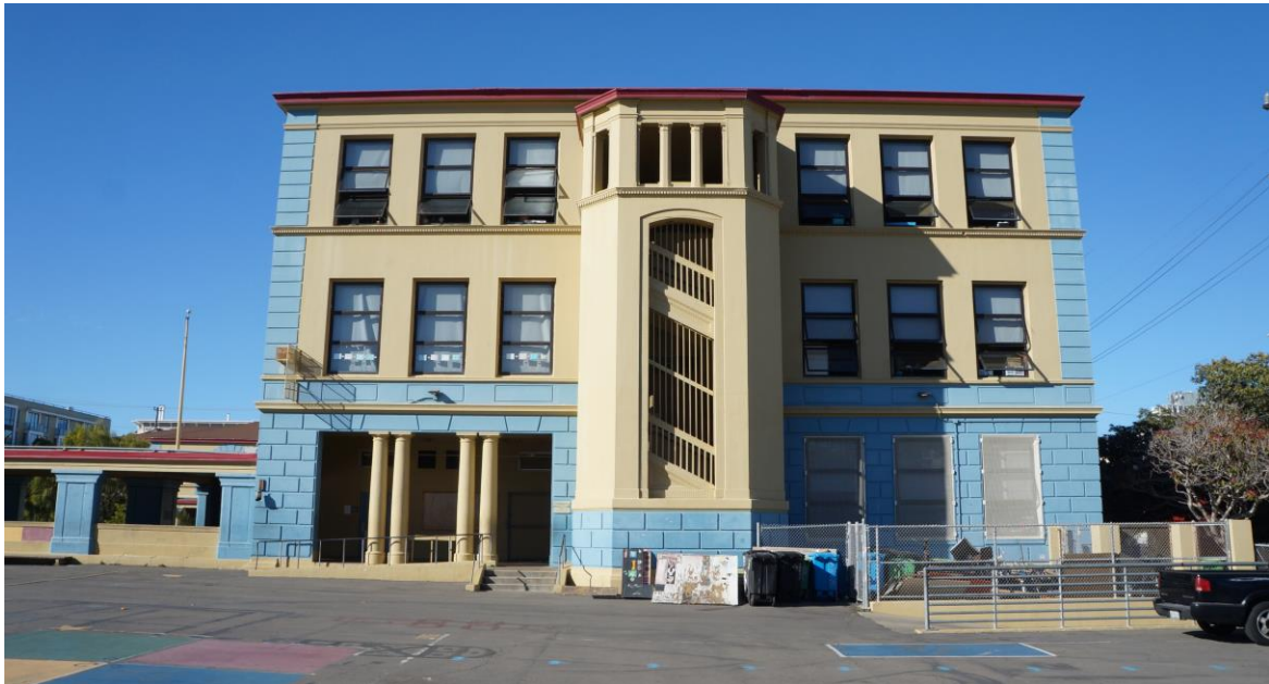
South façade of classroom wing, looking north. Knapp Architects 2022.
