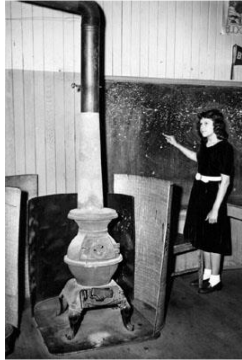
Interior of old Horace Mann School. San Francisco Public Library.
