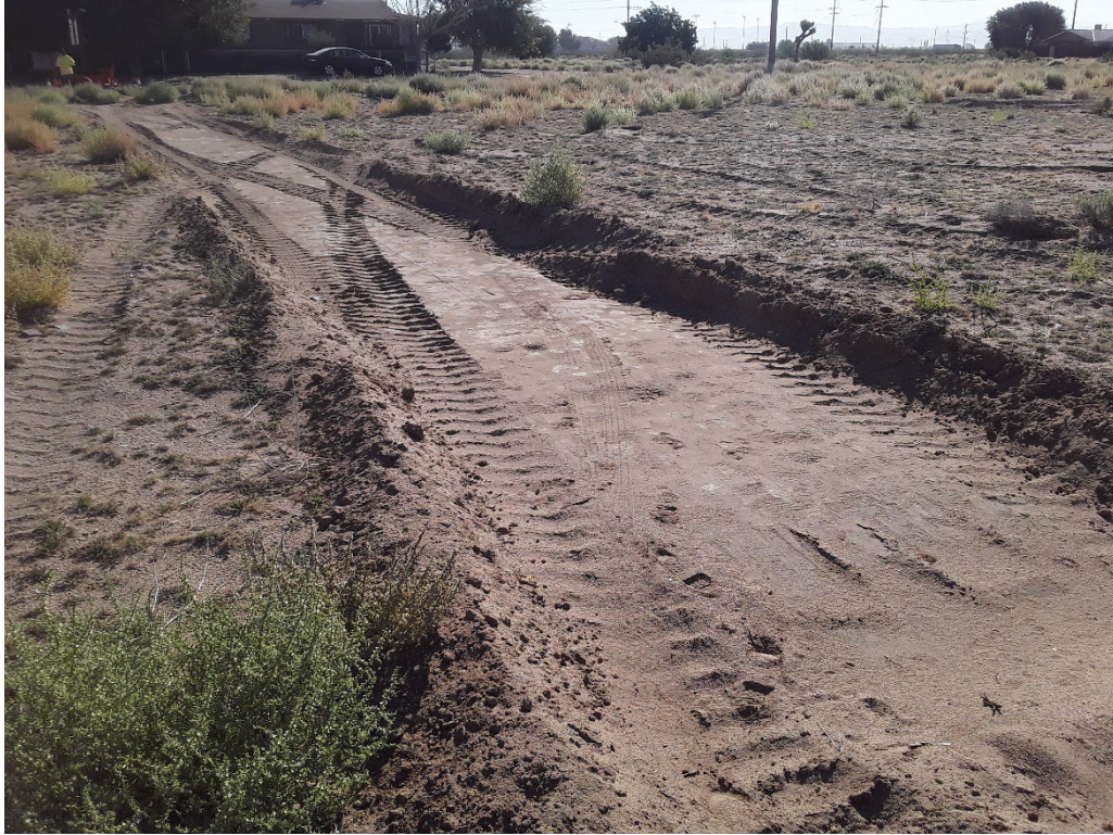
Heavy equipment cut. View to east.
