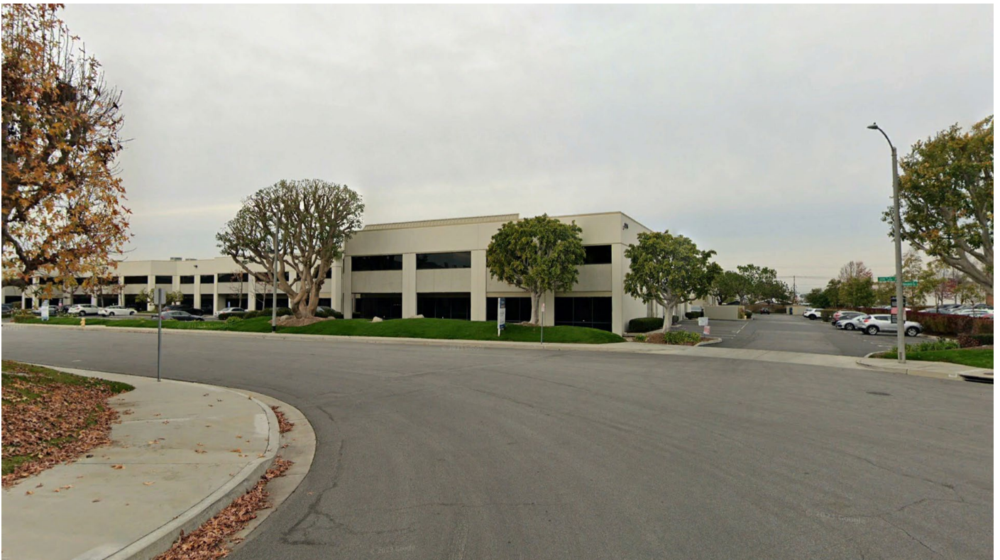
View of the southeast entrance from 205th St and Amapola Ave.
