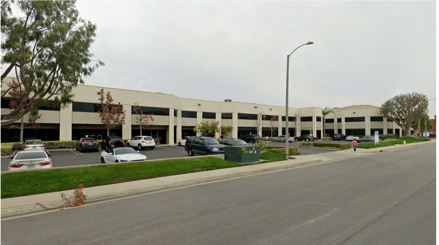
View of an existing structure from 205th St.
