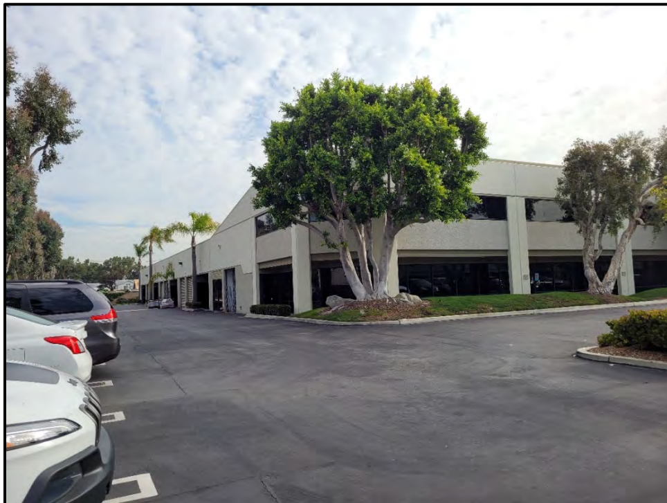
Plate 3.2-4: Overview from the southwest corner of the project, facing northeast.
