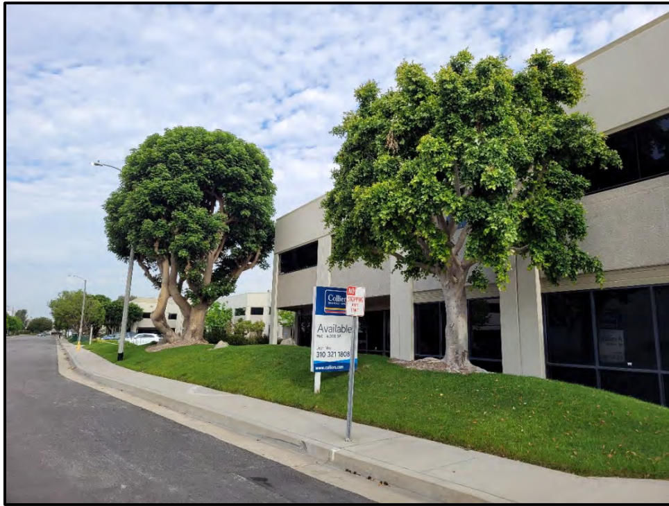
Plate 3.2-1: Overview from the southeast corner of the project, facing west.
