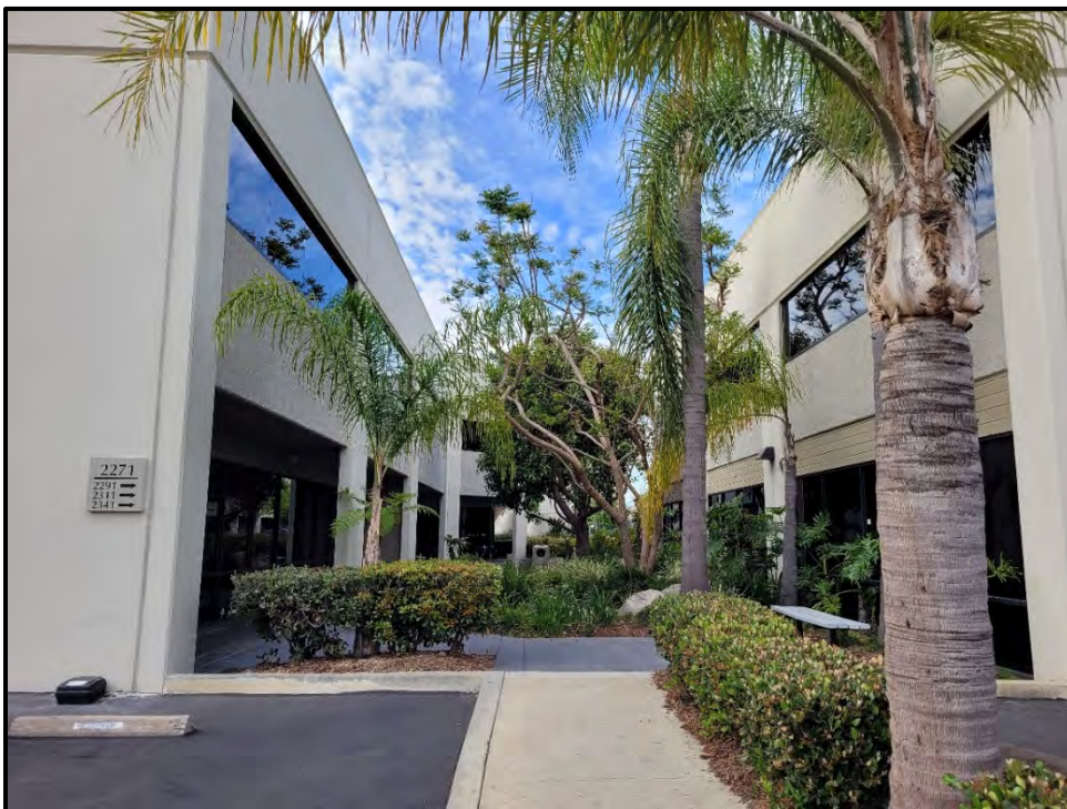
Plate 3.2–6: An example of introduced landscaping between buildings within the project, facing south.
